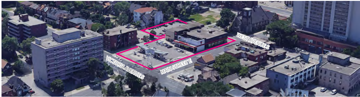
Figure 2. Site and the surrounding context area looking southwest (Google Earth 2023; annotated by ERA).
