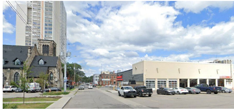
Figure 4 View From West Ave S Looking North
