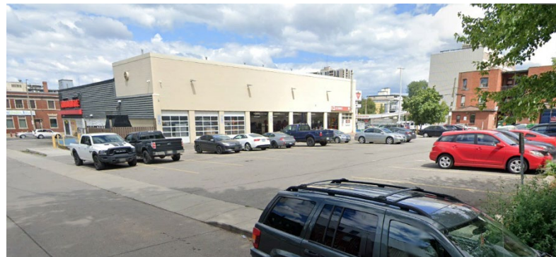
Figure 5 View From West Ave S and Laneway Looking West
