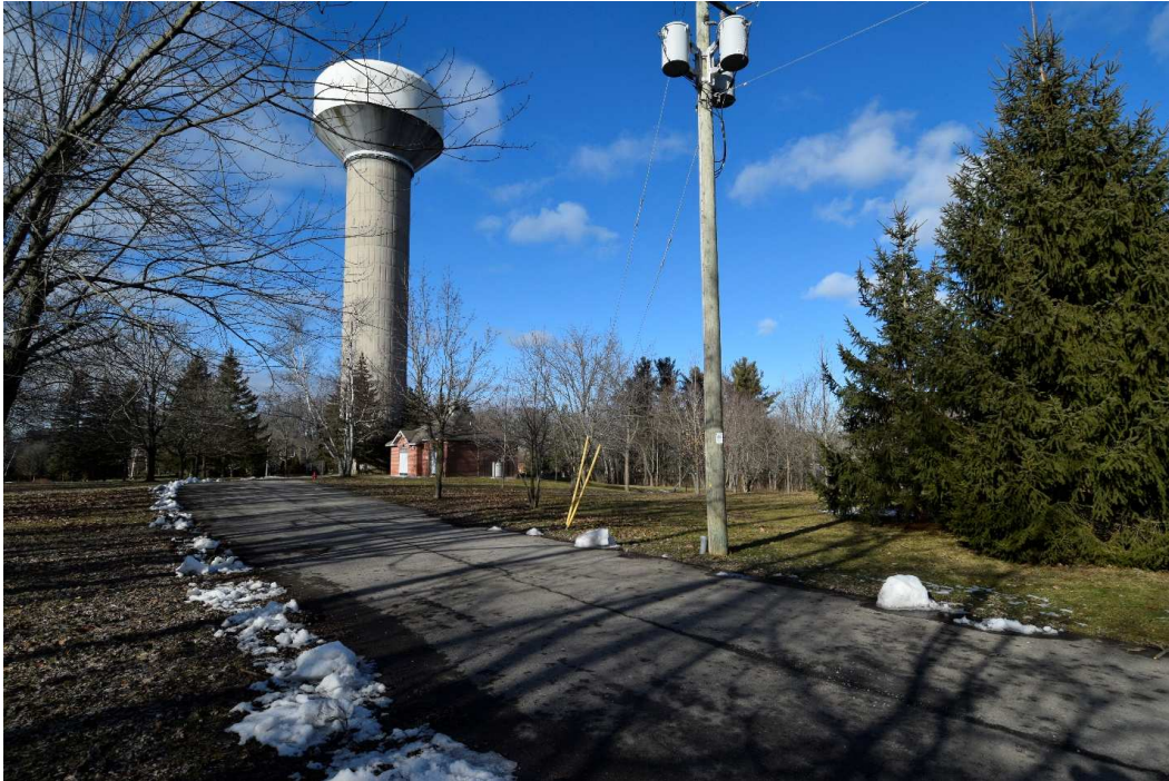
FIGURE 12: EXISTING WATER TOWER AND ASSOCIATED SURFACE INFRASTRUCTURE AT TOWER PARK, OPTION A IS TO THE RIGHT OF EXISTING TOWER
