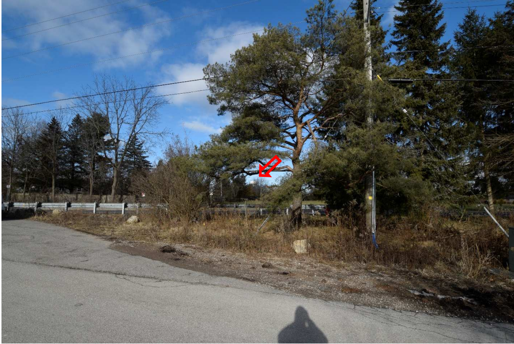
FIGURE 10: LOOKING NORTH FROM TERMINUS OF WILLIAM STREET TOWARDS TOWER PARK, RED ARROW INDICATES EXISTING WATER TOWER
