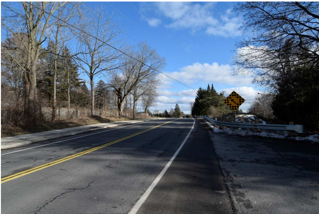
FIGURE 9: LOOKING SOUTHEAST DOWN CENTRE ROAD, WILLIAM STREET AND OPTION B ARE LOCATED TO THE RIGHT OF IMAGE
