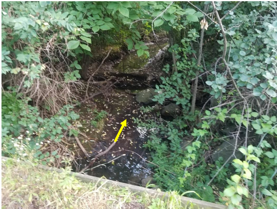
No bed scour was noted downstream of the Fruitland Road culvert.
