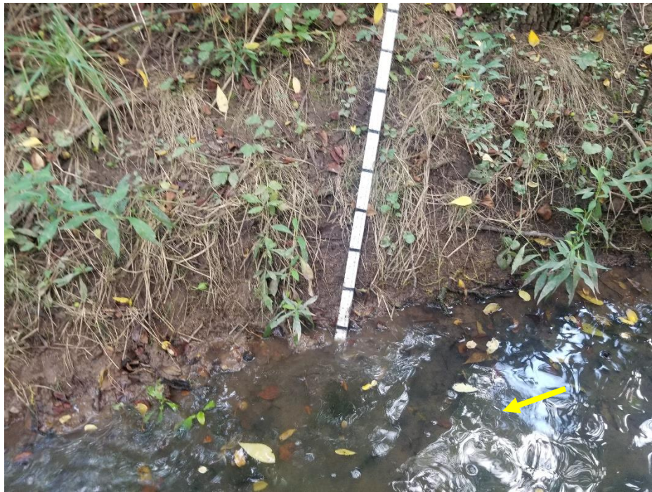
Bank materials across the entire reach are characterized by silty clay. Occasional tree roots were observed, but the bottom third of the bank is typically exposed.
