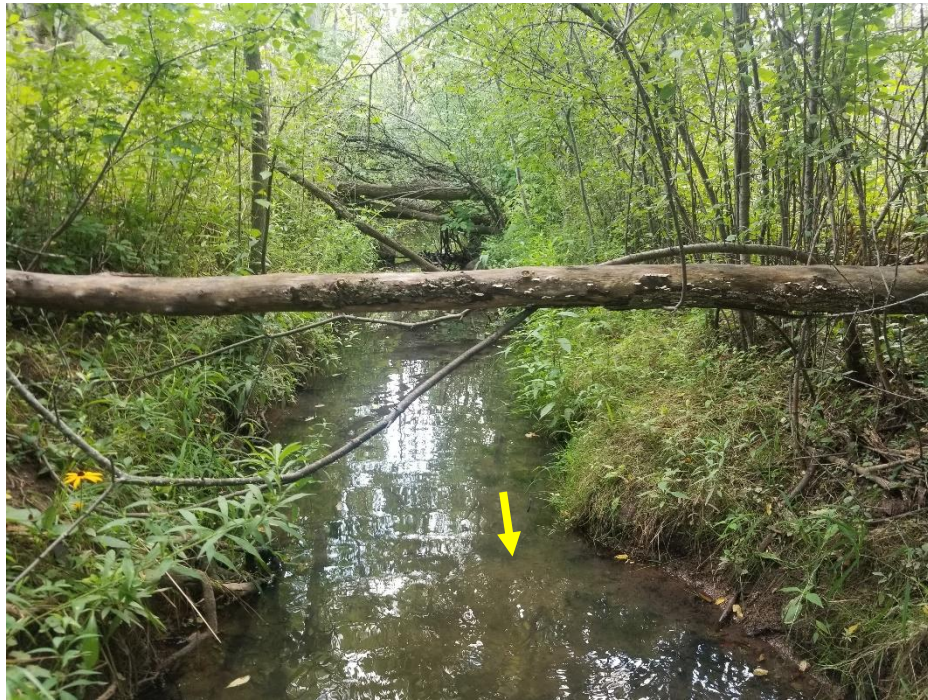
Reach WC5 has a predominantly trapezoidal channel shape throughout the study area. Minimal flow velocities were observed during the assessment.
