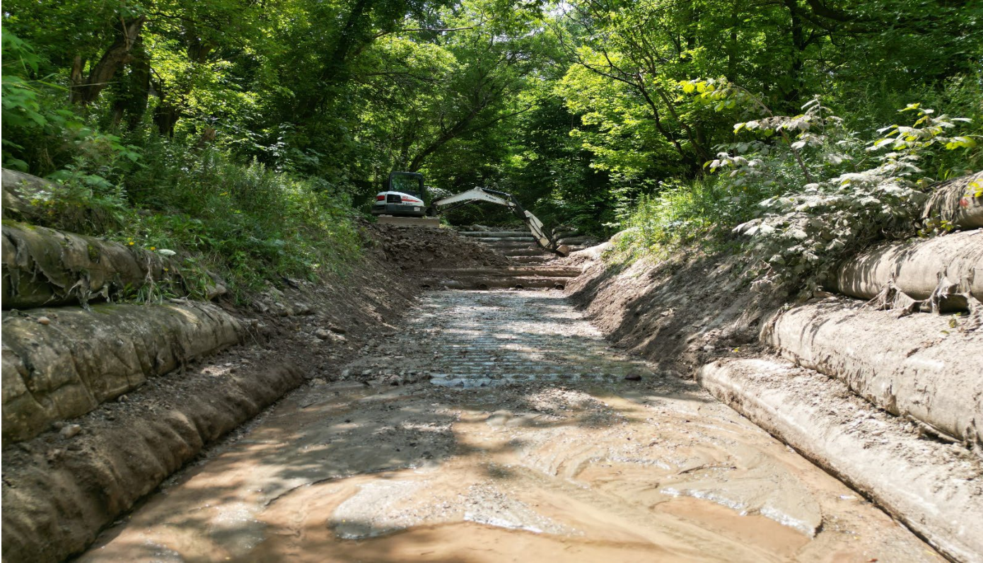
Sydenham Creek Retaining Wall:
