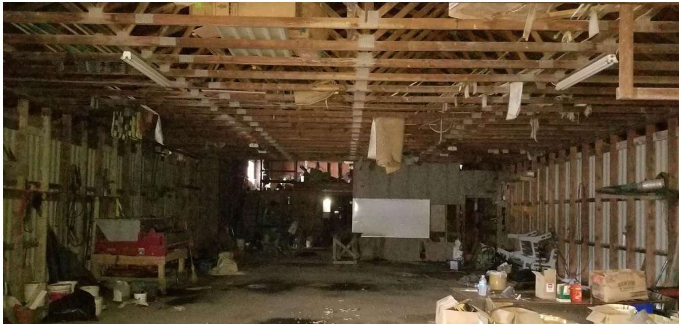
Figure 30: 555 Glanaster Road: Exposed wood frame and roof trusses of the outbuilding
