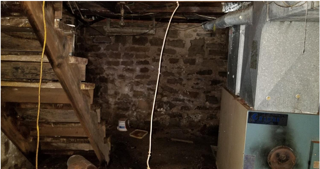
Figure 74: 9751 Twenty Road West: Wood stairs leading down to the basement
