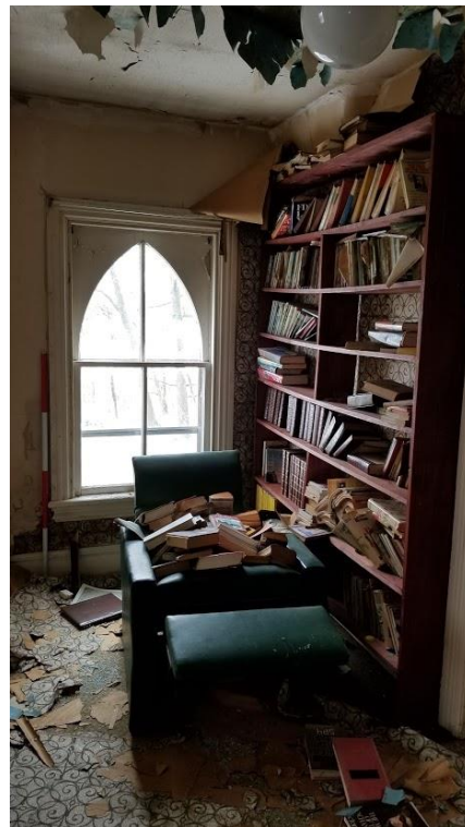
Figure 65: 9751 Twenty Road West: Pointed window in the central hallway
