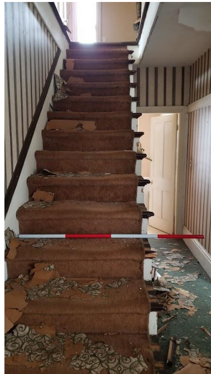
Figure 57: 9751 Twenty Road West: Staircase leading to the second storey
