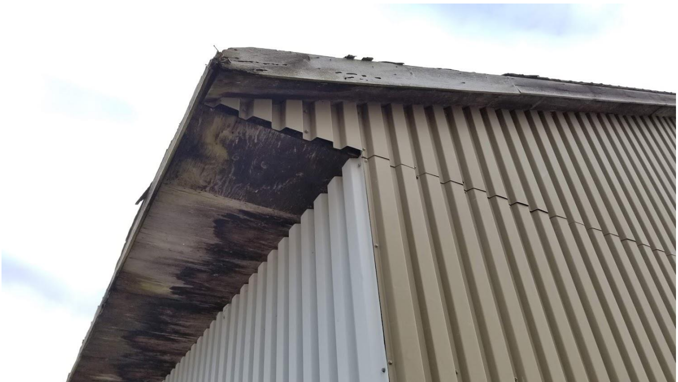
Figure 29: 555 Glancaster Road: Wood eaves at the outbuilding
