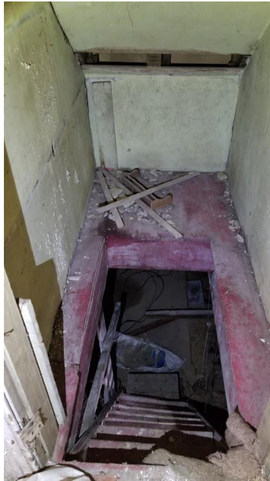
Figure 112: 9285 Twenty Road West: Wood stairs leading to the basement
