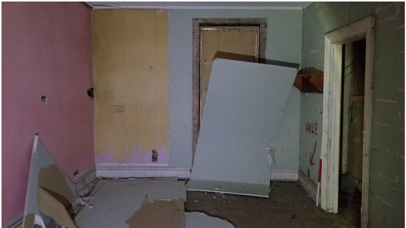
Figure 107: 9285 Twenty Road West: Room at the southwest corner of the house
