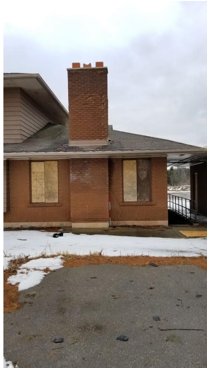
Figure 18: 555 Glancaster Road: Three stack brick chimney on the east façade
