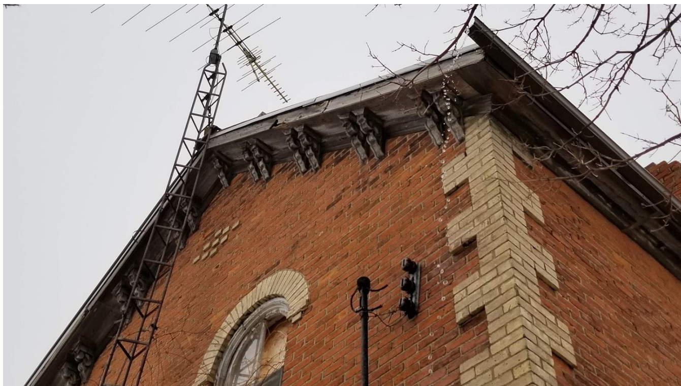
Figure 88: 9285 Twenty Road West: Yellow brick detailing at the centre of the gable roof
