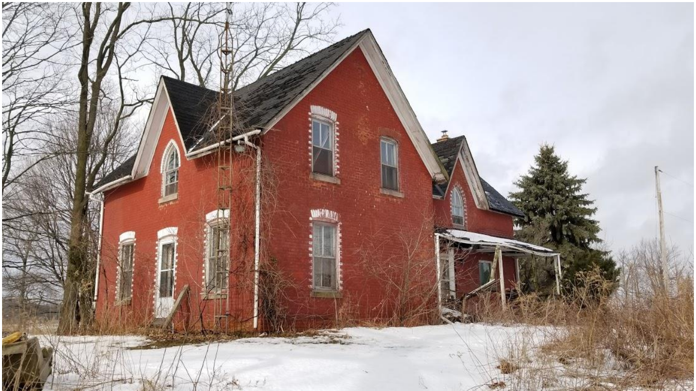
Figure 33: 9751 Twenty Road West: South and east façades
