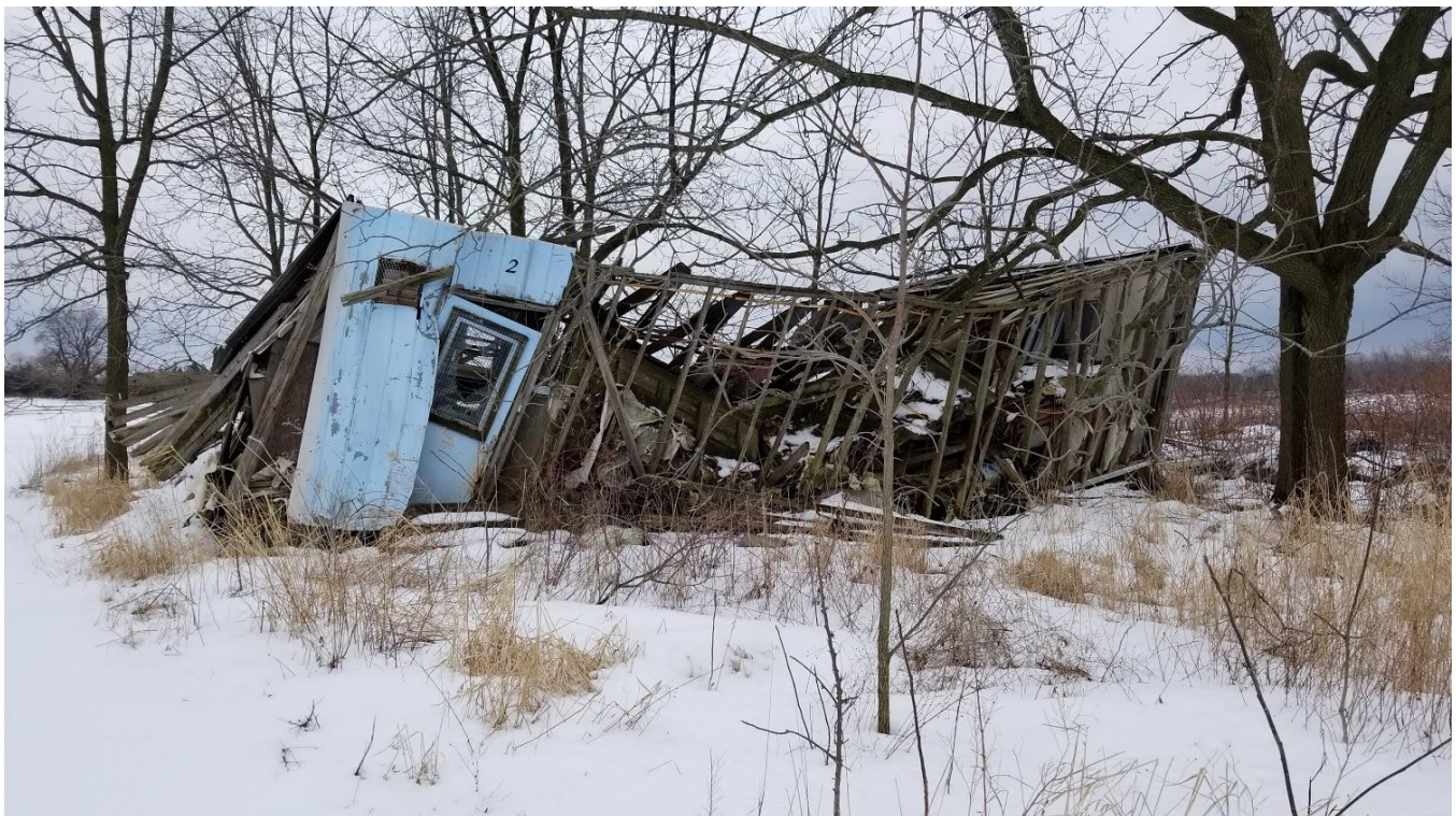
Figure 49: 9751 Twenty Road West: Remnants of an outbuilding to the northeast of the house
