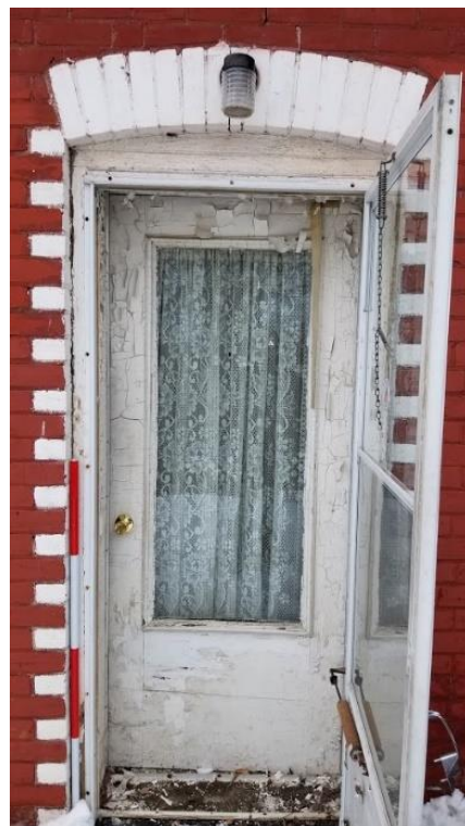
Figure 43: 9751 Twenty Road West: Main entrance on the west facade with painted soldier voussoirs
