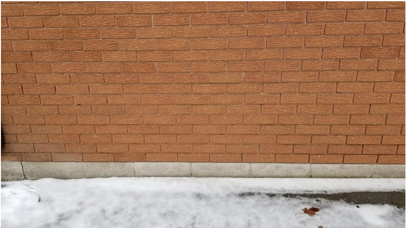
Figure 17: 555 Glancaster Road: Concrete foundation and red stretcher brick cladding
