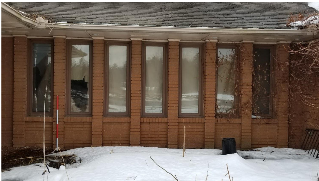
Figure 21: 555 Glancaster Road: Vertical rectangular windows on the south façade
