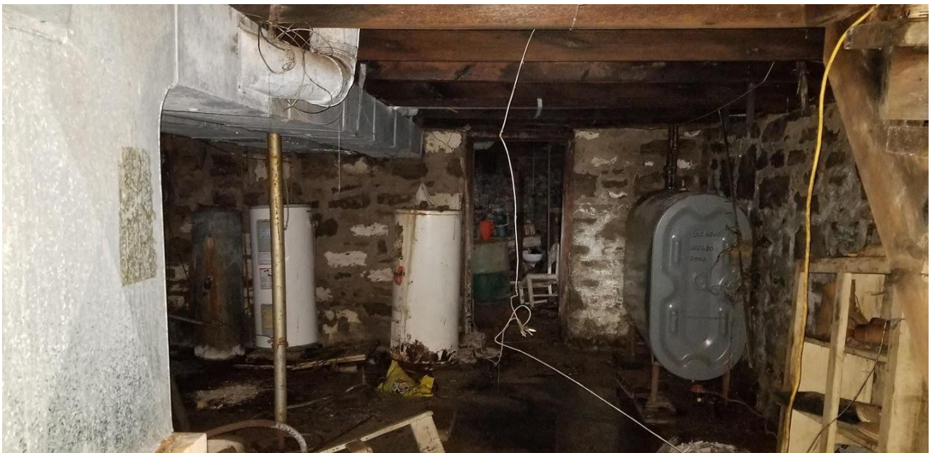
Figure 75: 9751 Twenty Road West: Basement facing south
