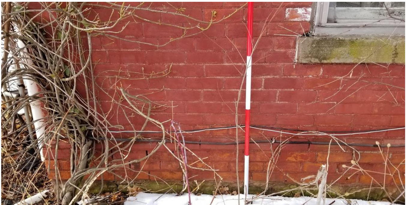
Figure 37: 9751 Twenty Road West: Coursed rubble foundation with red common brick cladding
