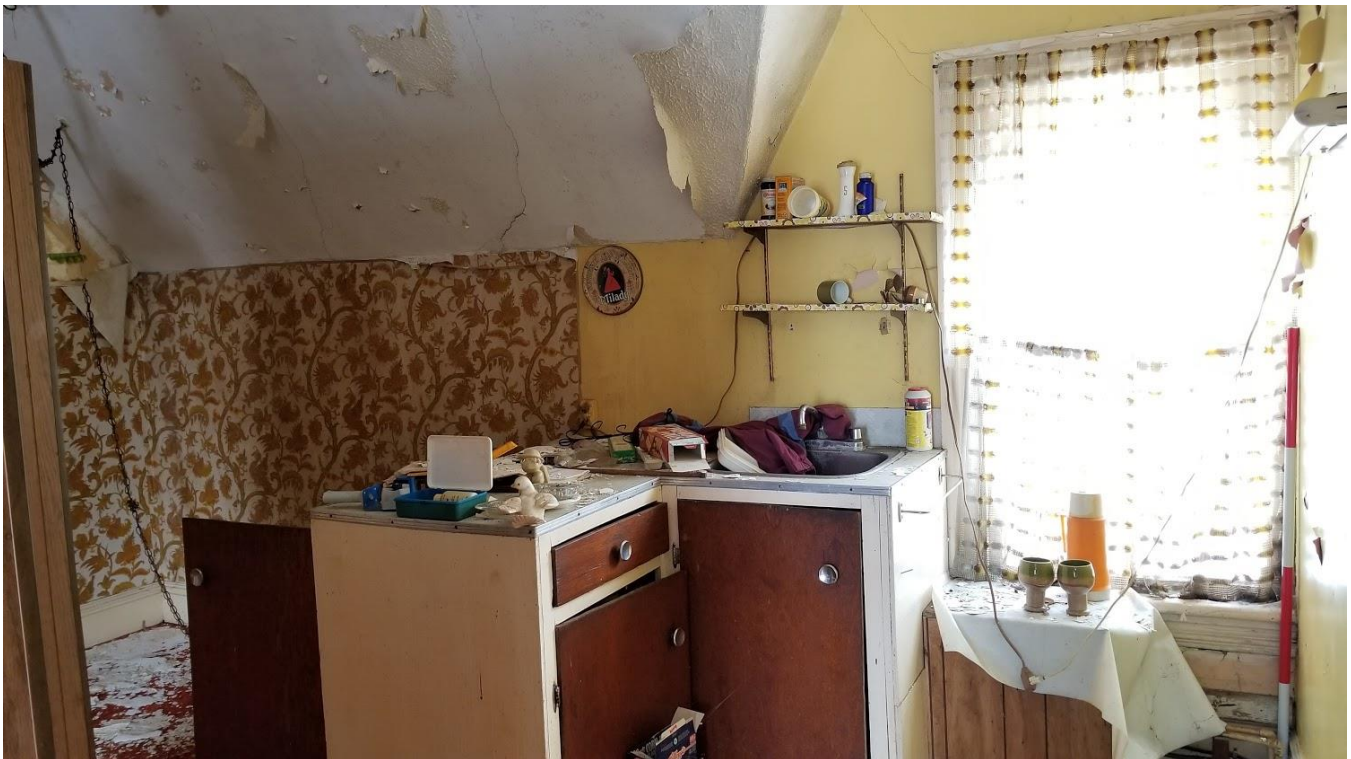
Figure 73: 9751 Twenty Road West: Large room facing west
