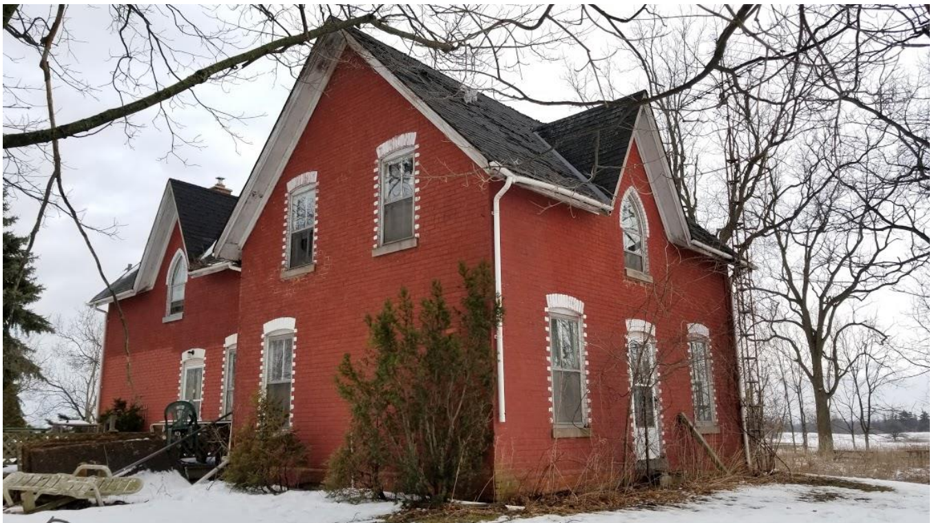
Figure 36: 9751 Twenty Road West: West and south façades
