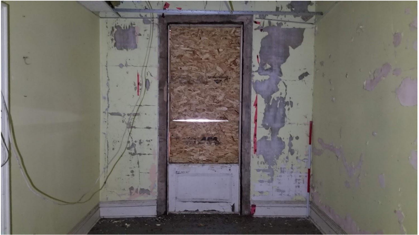
Figure 110: 9285 Twenty Road West: Bedroom at the southeast corner of the house
