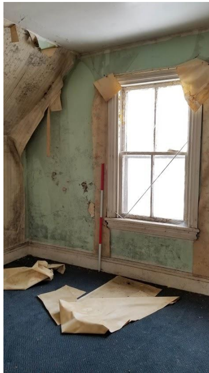
Figure 66: 9751 Twenty Road West: Room to the east of the central hallway
