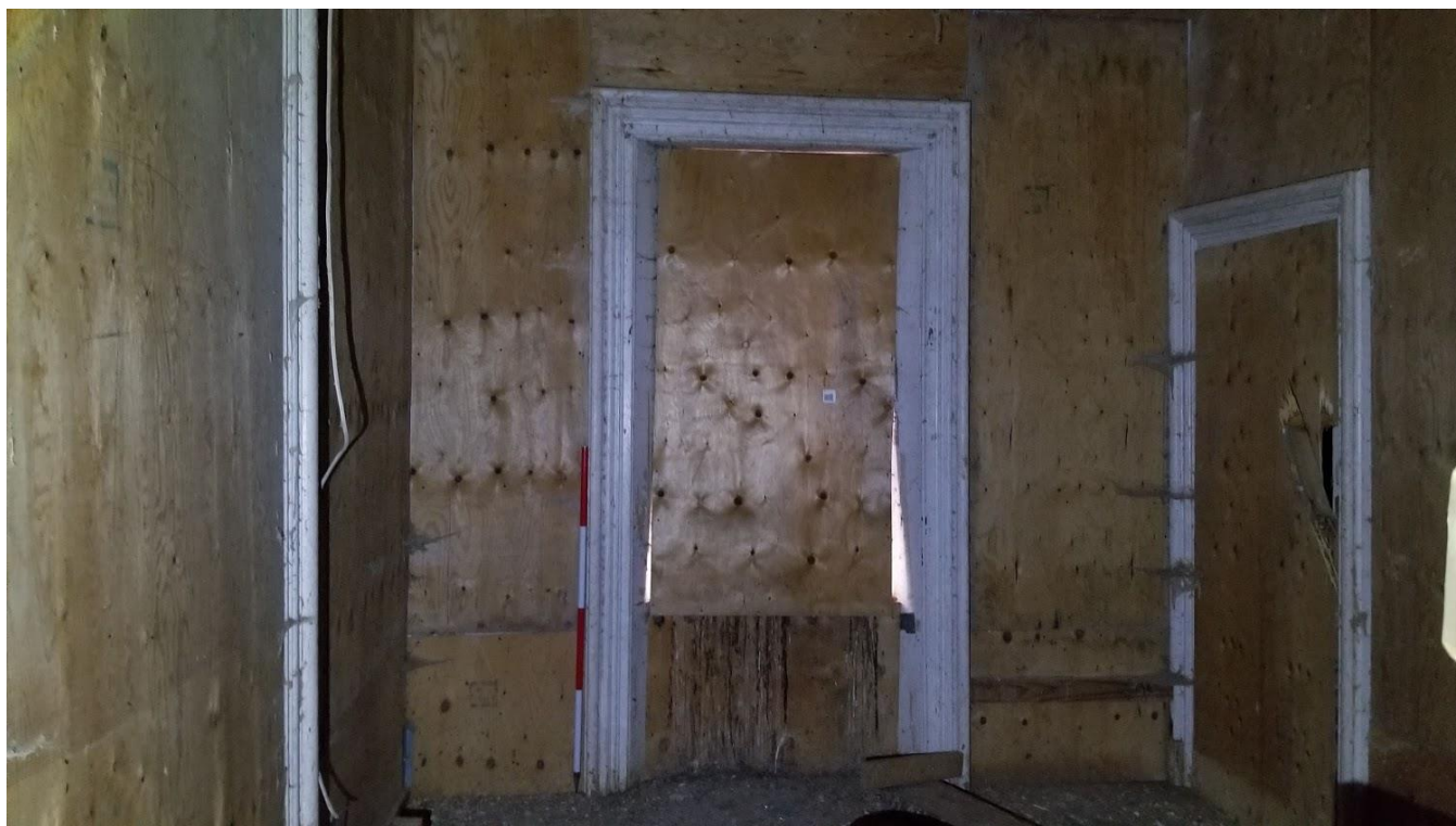
Figure 101: 9285 Twenty Road West: Northeast corner room, clad in plywood
