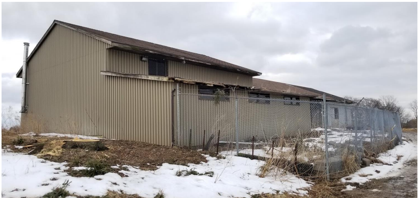
Figure 25: 555 Glancaster Road: West and south façades of the outbuilding
