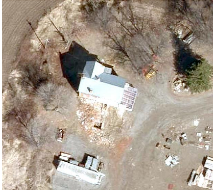
Figure 3.0: Aerial Photo circa 2010 (Source: City of Hamilton Mapping) Featuring demolished south addition and new east shed addition
