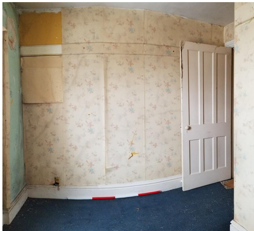
Figure 67: 9751 Twenty Road West: Room to the east of the central hallway
