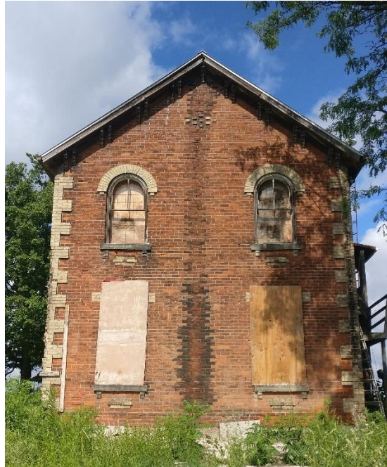
Figure 5.0: East Façade of Building
