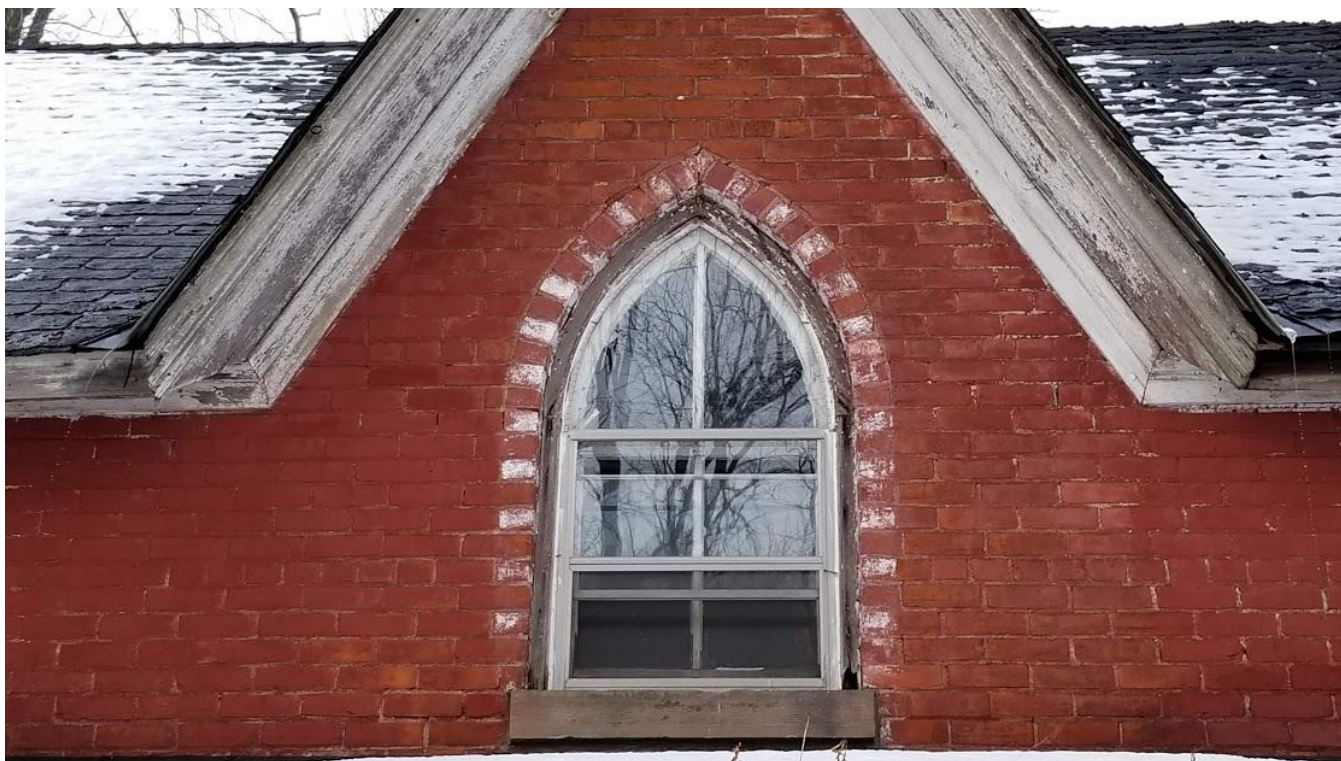
Figure 40: 9751 Twenty Road West: Pointed window at the centre of cross gable with bush hammered lug sill
