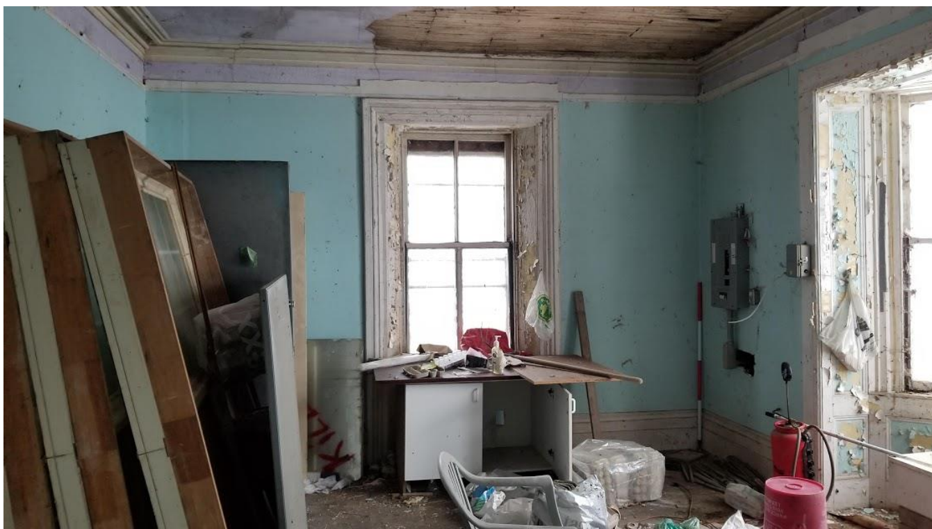
Figure 98: 9285 Twenty Road West: Room at the northwest corner of the house with crown moulding, wide baseboards and decorative trim around doors and windows
