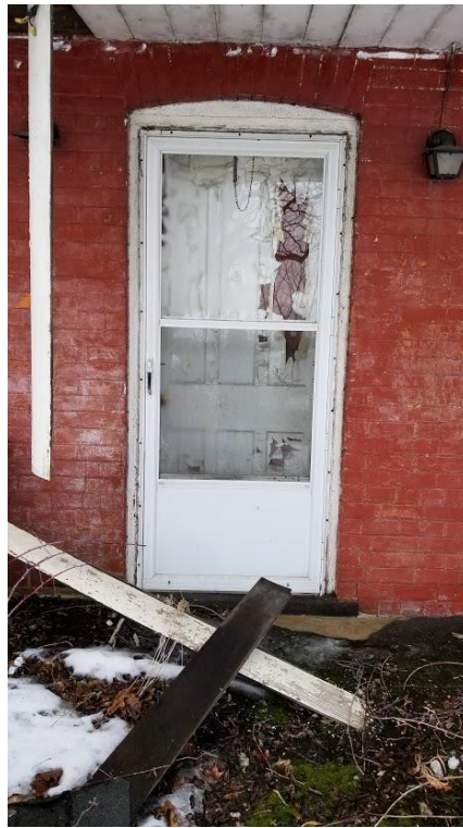
Figure 44: 9751 Twenty Road West: Single-leaf entrance on the east façade
