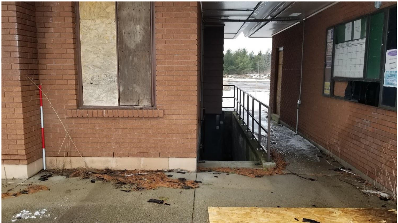
Figure 19: 555 Glancaster Road: Stairs leading to the basement
