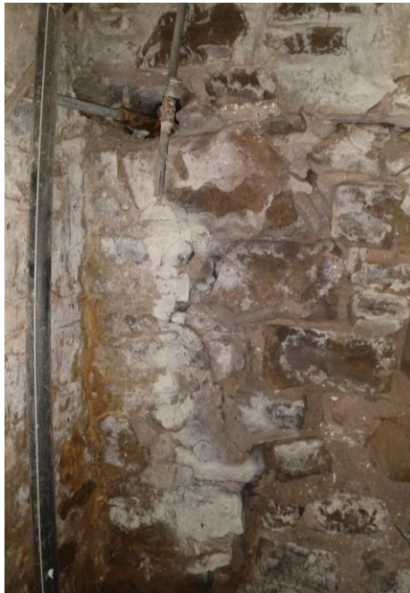
Figure 16.0: Typical Rubble Stone Foundation Wall
