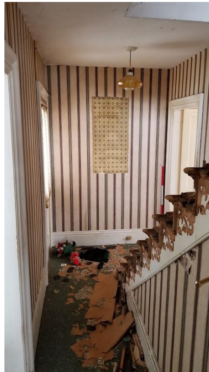
Figure 55: 9751 Twenty Road West: Hallway
