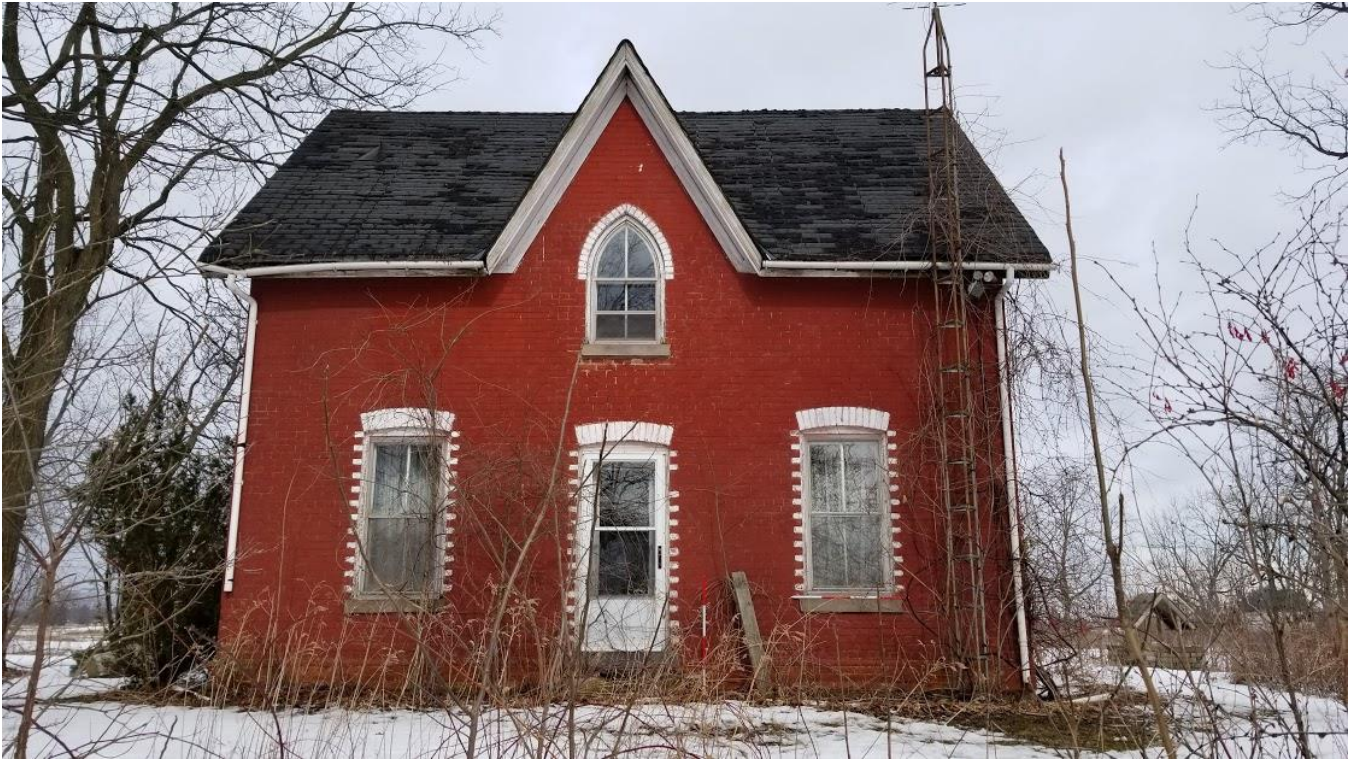
Figure 32: 9751 Twenty Road West: South façade
