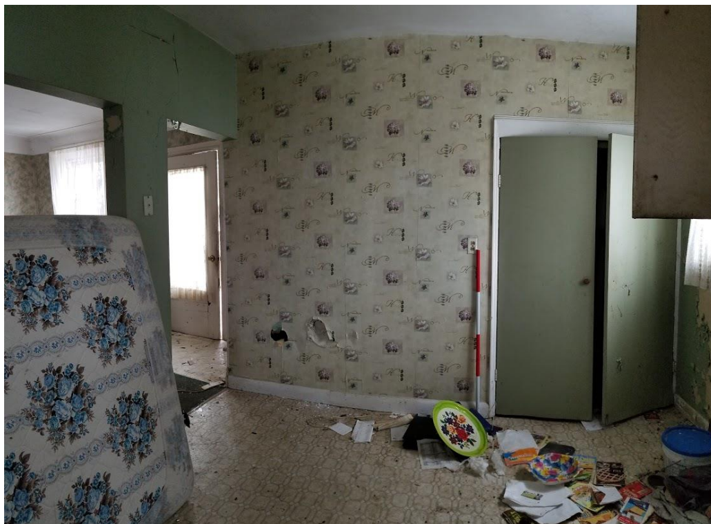
Figure 54: 9751 Twenty Road West: Former kitchen facing west
