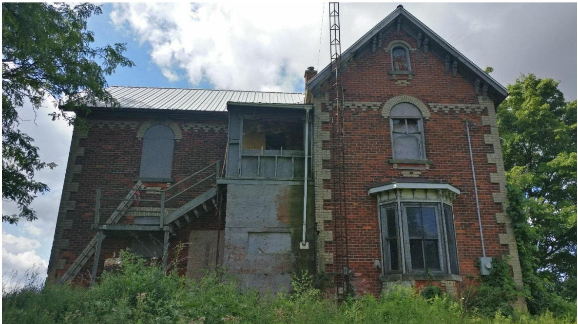
Figure 4.0: North Façade of Building Featuring exterior stair access to 2 nd floor
