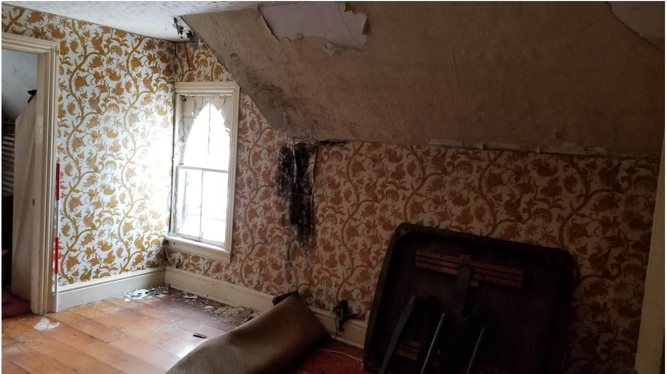
Figure 72: 9751 Twenty Road West: Large room facing east towards the cross gable
