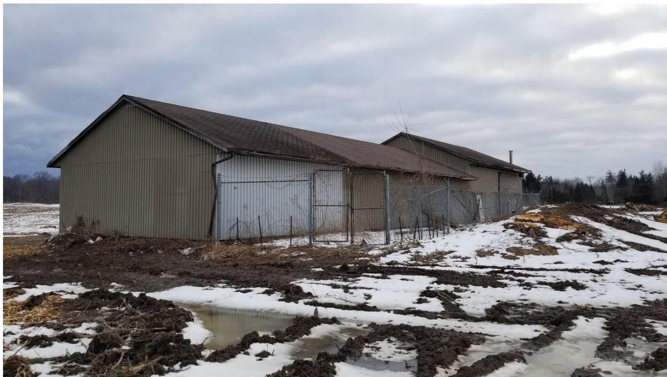
Figure 27: 555 Glanaster Road: North and east façades of the outbuilding
