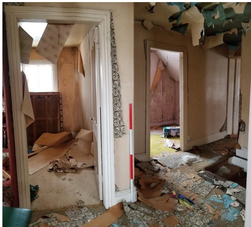
Figure 63: 9751 Twenty Road West: Central hallway
