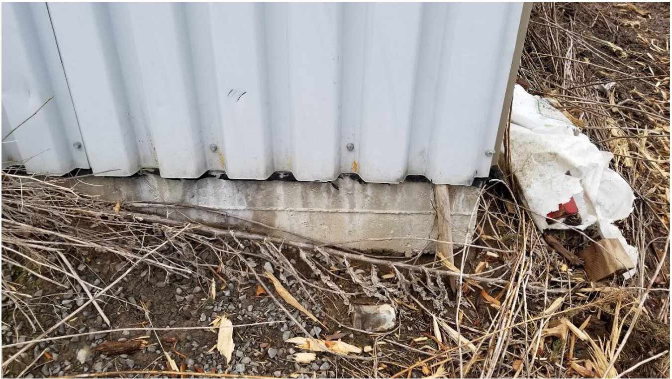
Figure 28: 555 Glancaster Road: Concrete foundation of the outbuilding
