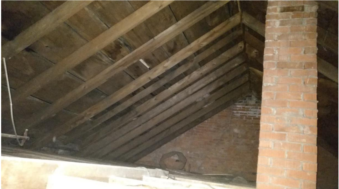
Figure 21.0: Typical Roof Framing
