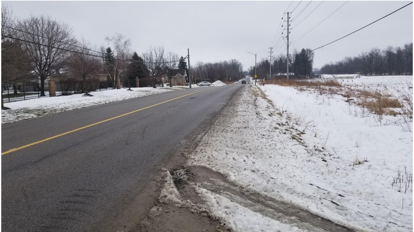
Figure 8: Twenty Road West facing east from 9285 Twenty Road West
