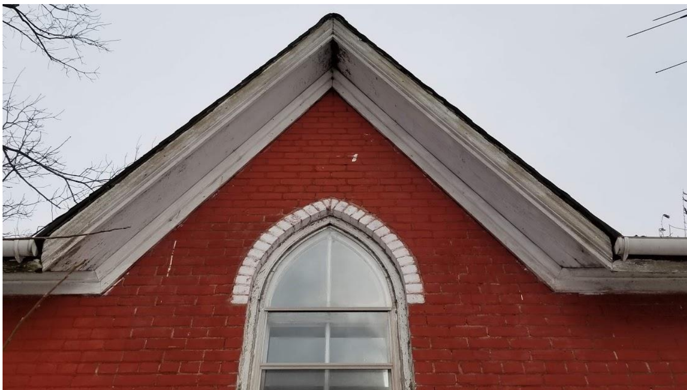
Figure 38: 9751 Twenty Road West: Centre gable on the south façade
