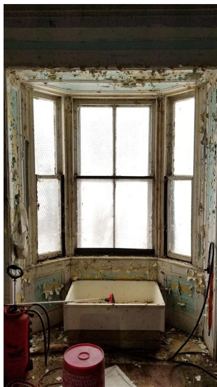
Figure 99: 9285 Twenty Road West: Bay window along the north façade wall
