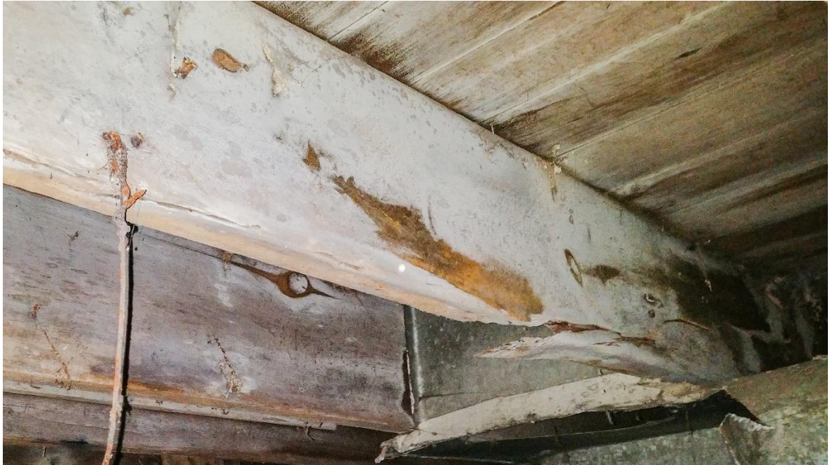
Figure 13.0: Typical Split Ground Level Floor Joist
