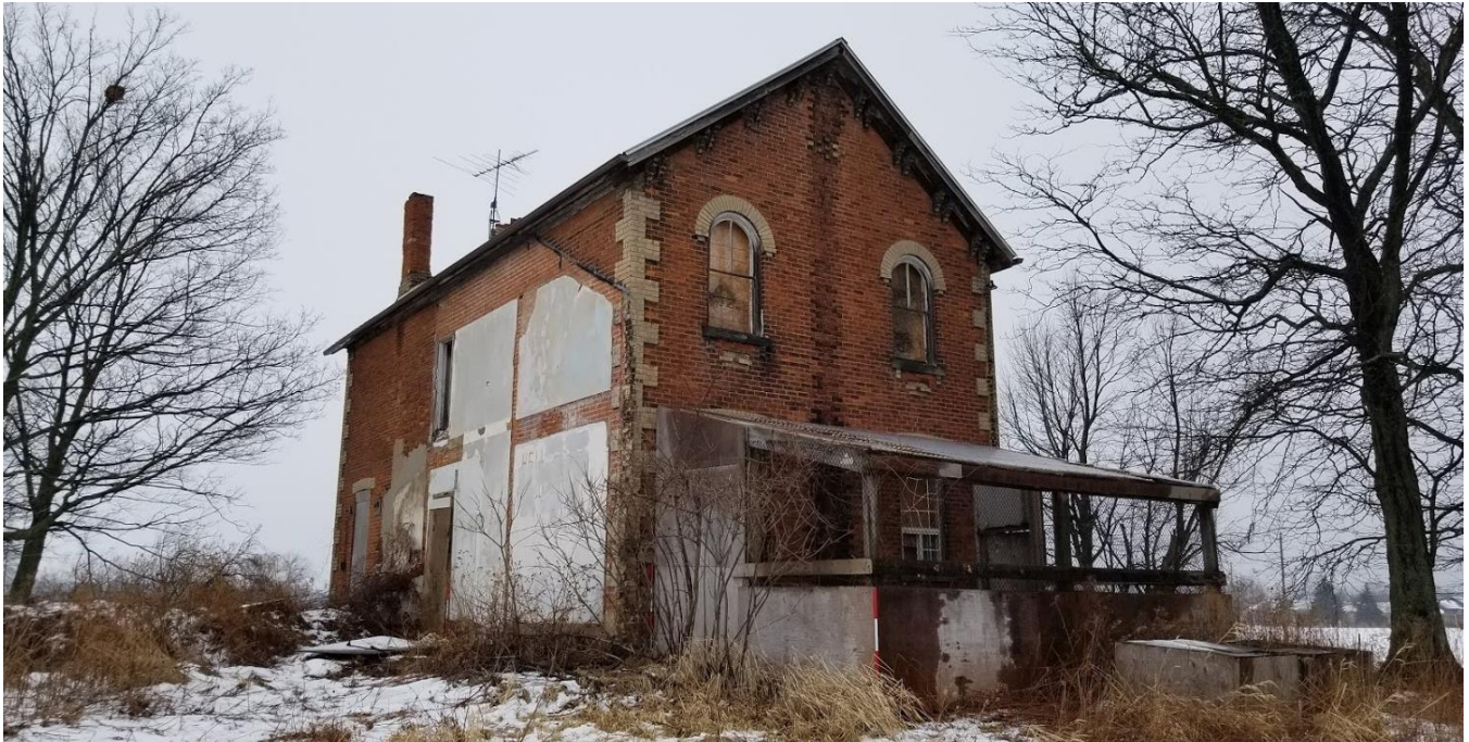
Figure 82: 9285 Twenty Road West: East and south façades
