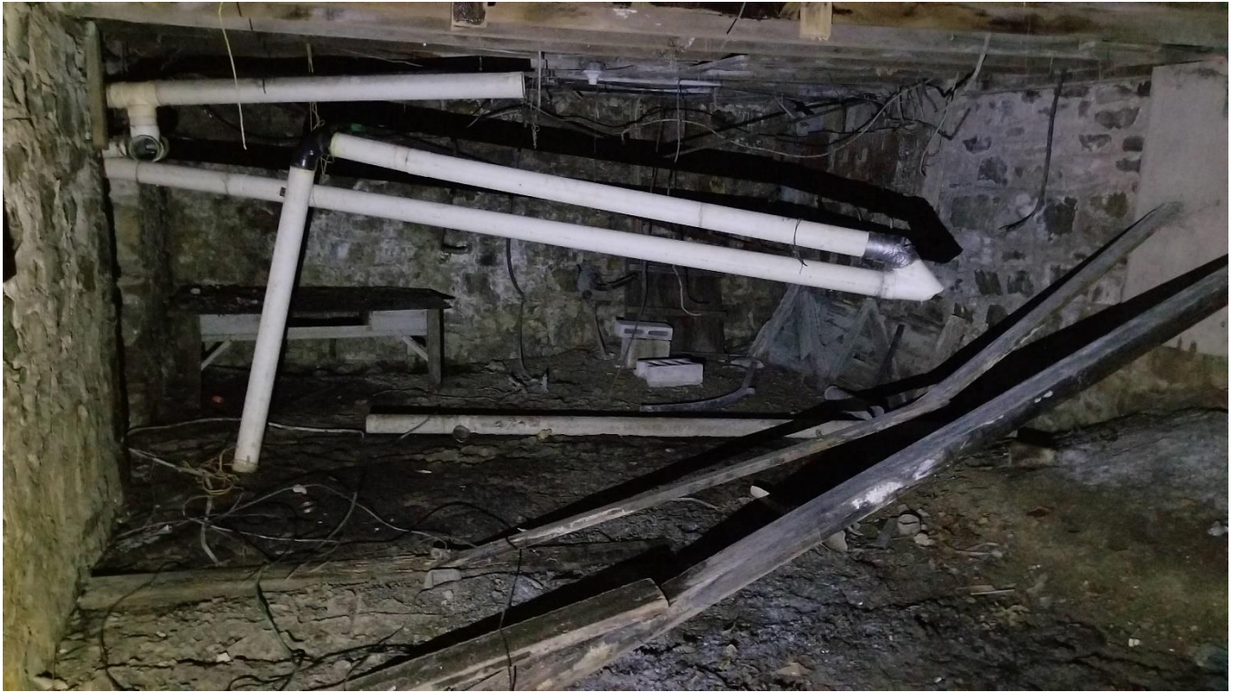
Figure 117: 9285 Twenty Road West: Large room to the west, facing south
