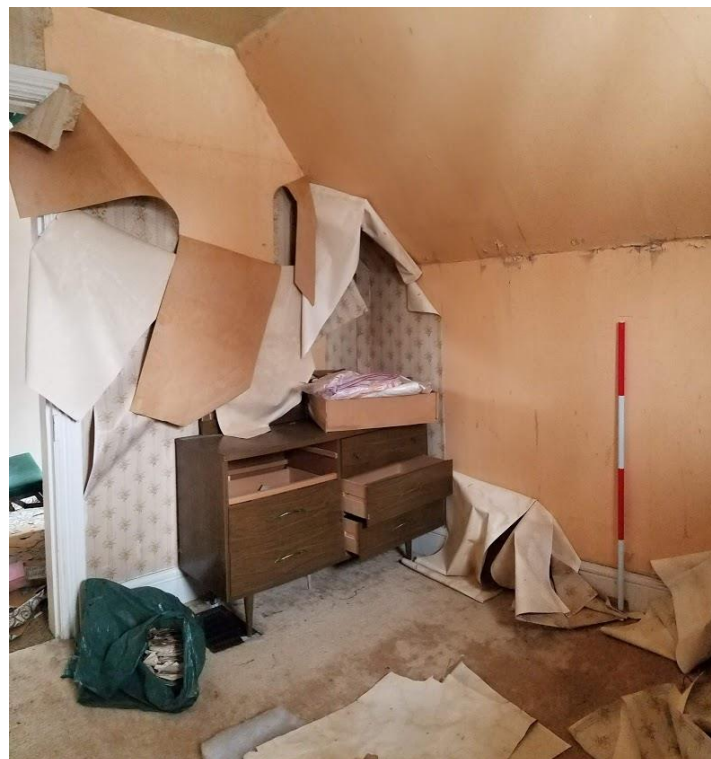
Figure 69: 9751 Twenty Road West: Southeast room
