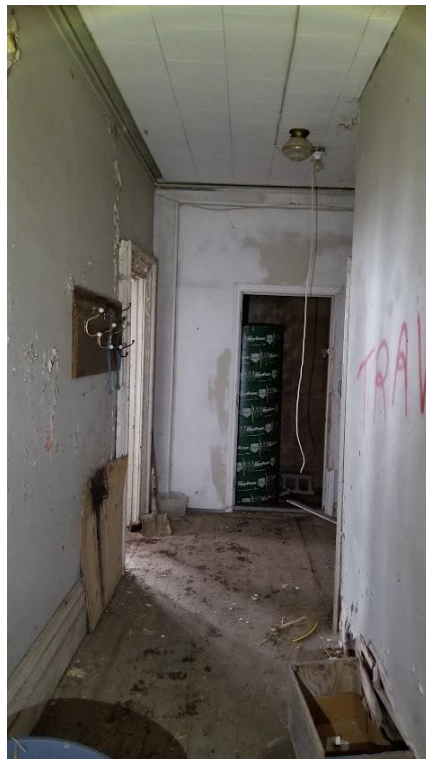
Figure 96: 9285 Twenty Road West: Central hallway facing towards the main entrance
