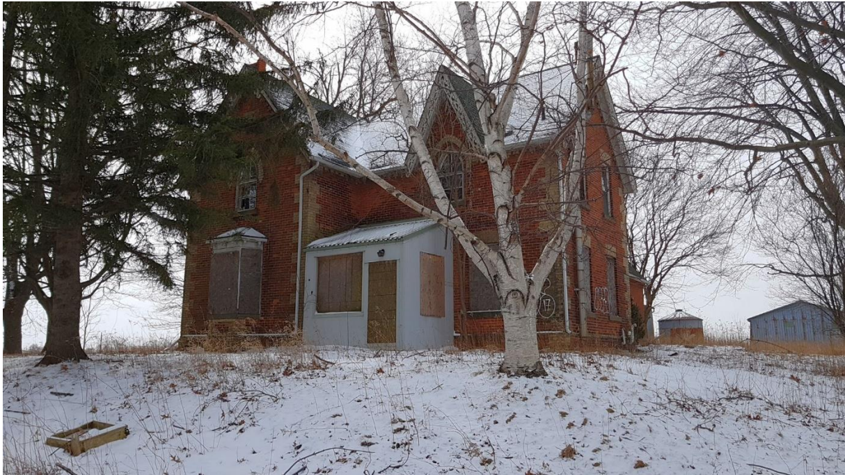
Figure 124: 9445 Twenty Road West (Golder 2018)
