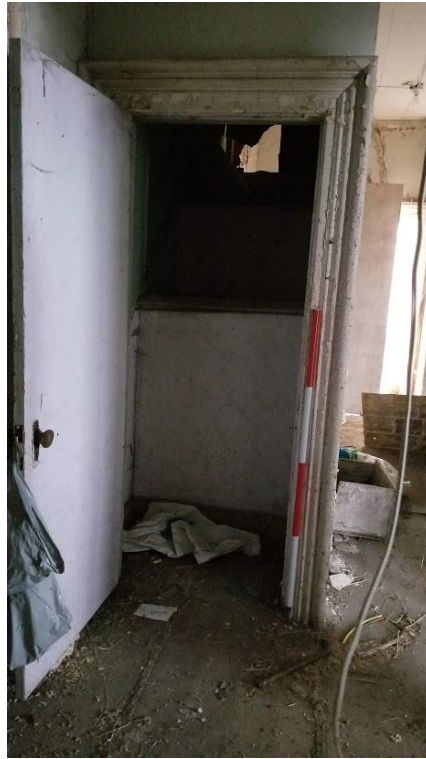
Figure 95: 9285 Twenty Road West: Staircase in the central hallway providing access to the second storey, which was blocked
