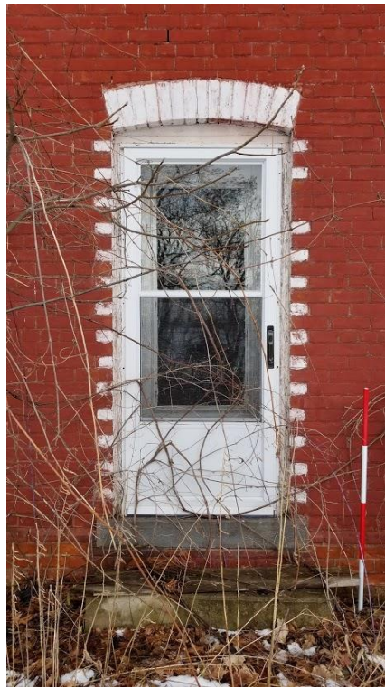
Figure 46: 9751 Twenty Road West: Entrance on the south facade
