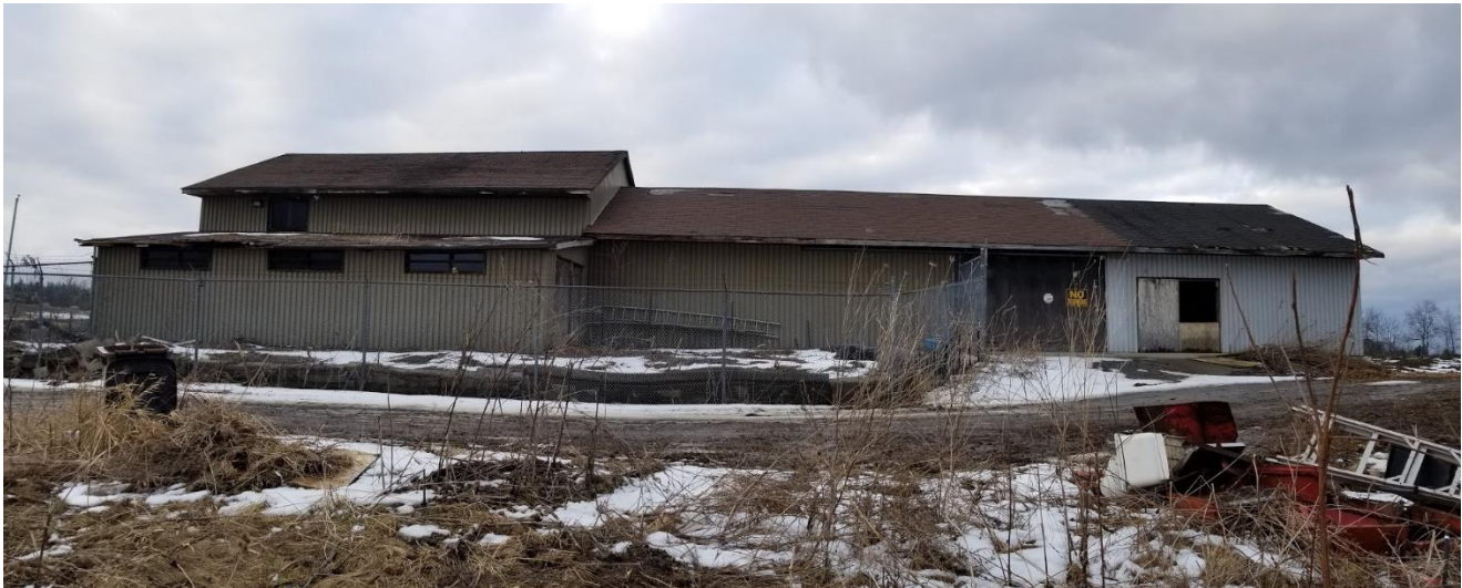
Figure 24: 555 Glancaster Road: South façade of the outbuilding
