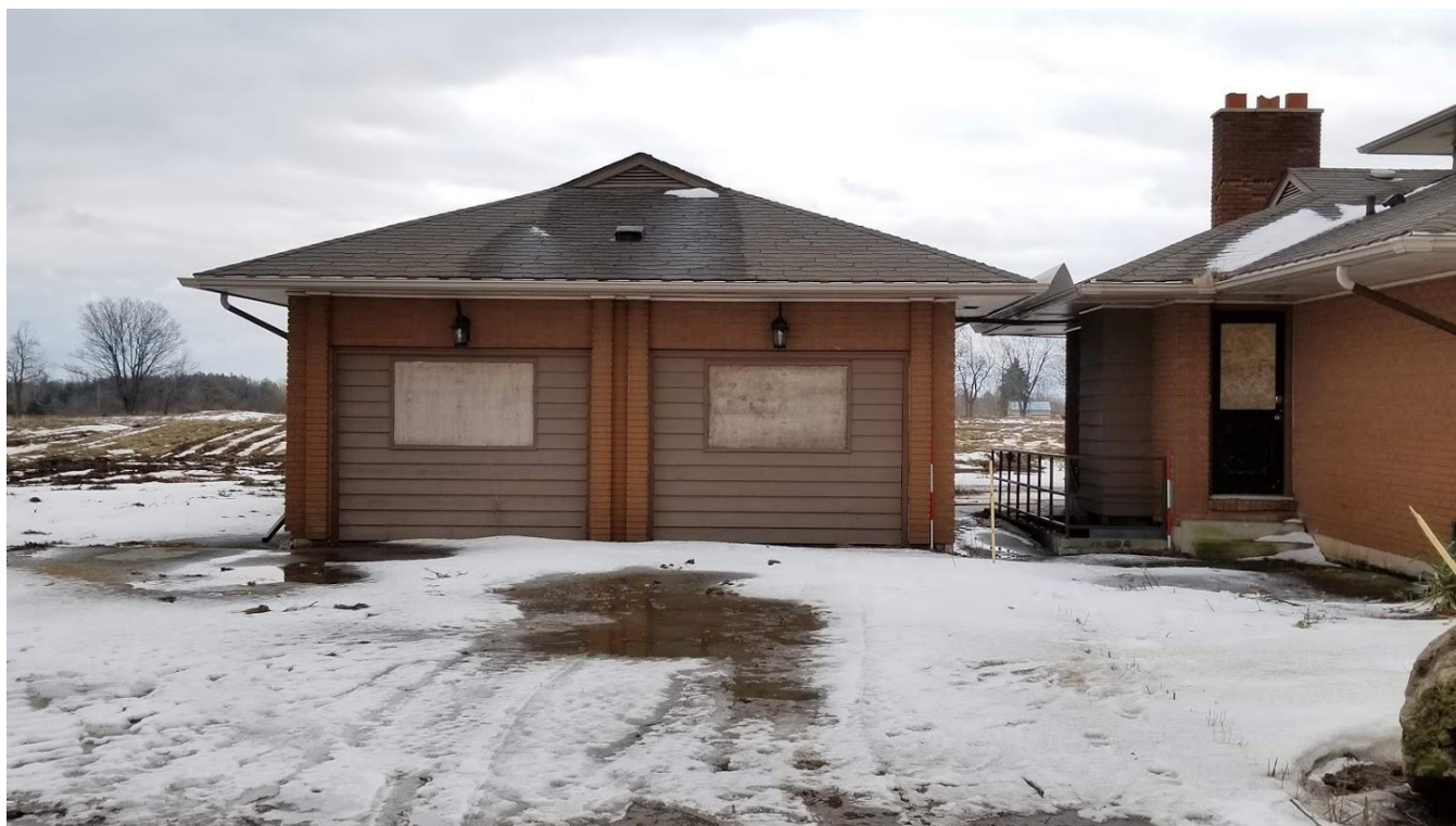
Figure 20: 555 Glancaster Road: Semi-detached double garage
