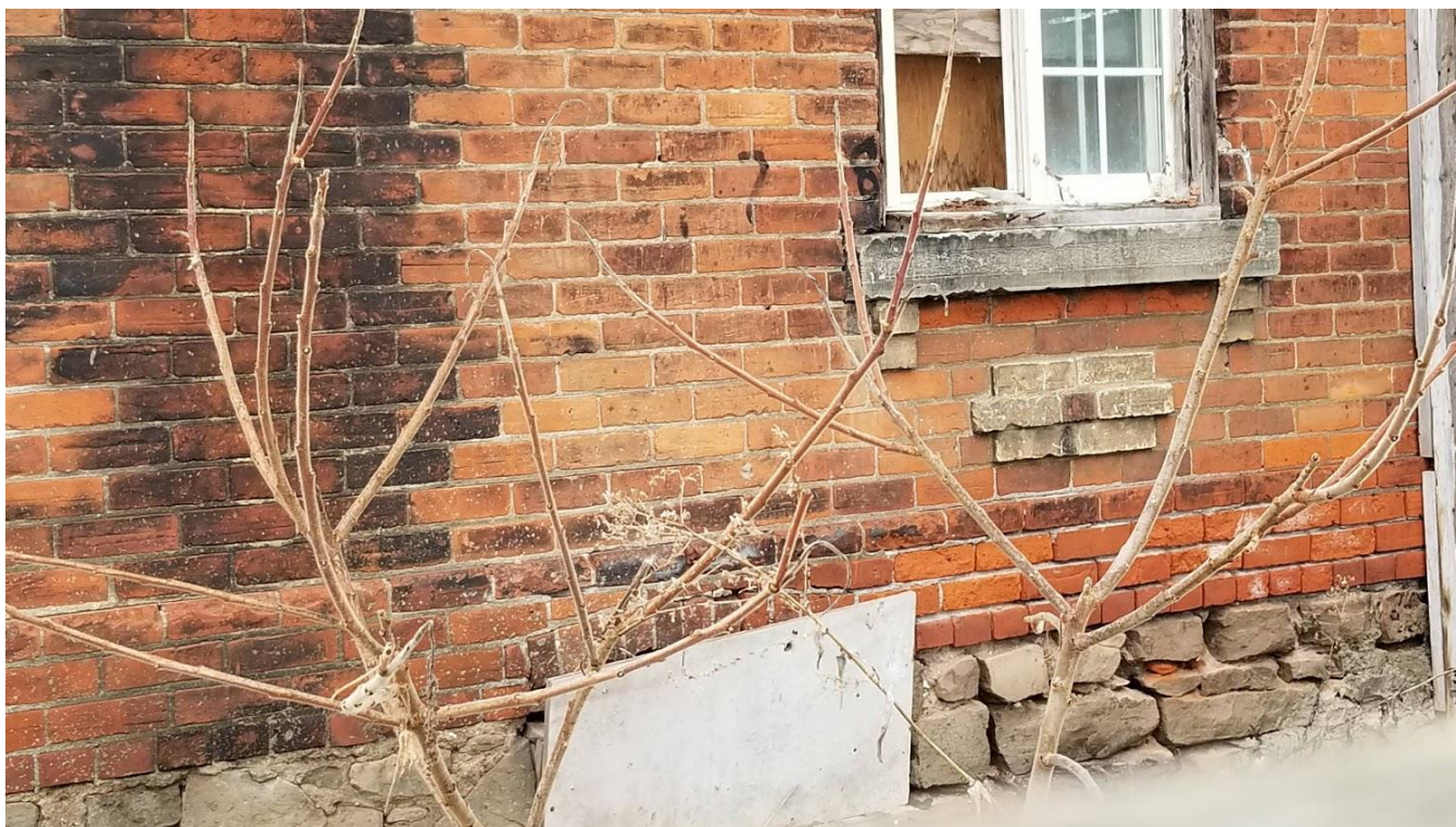
Figure 87: 9285 Twenty Road West: Yellow brick detailing underneath the windows
