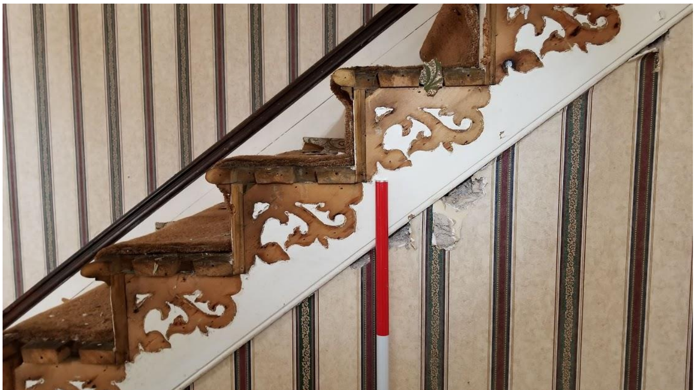
Figure 56: 9751 Twenty Road West: Staircase with railing and decorative trim removed
