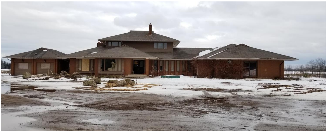
Figure 14: 555 Glancaster Road: West façade
