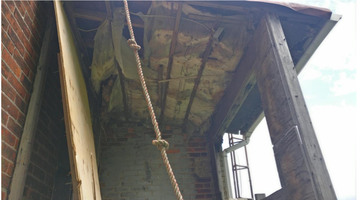
Figure 19.0: Exterior Stair Landing Roof Framing
