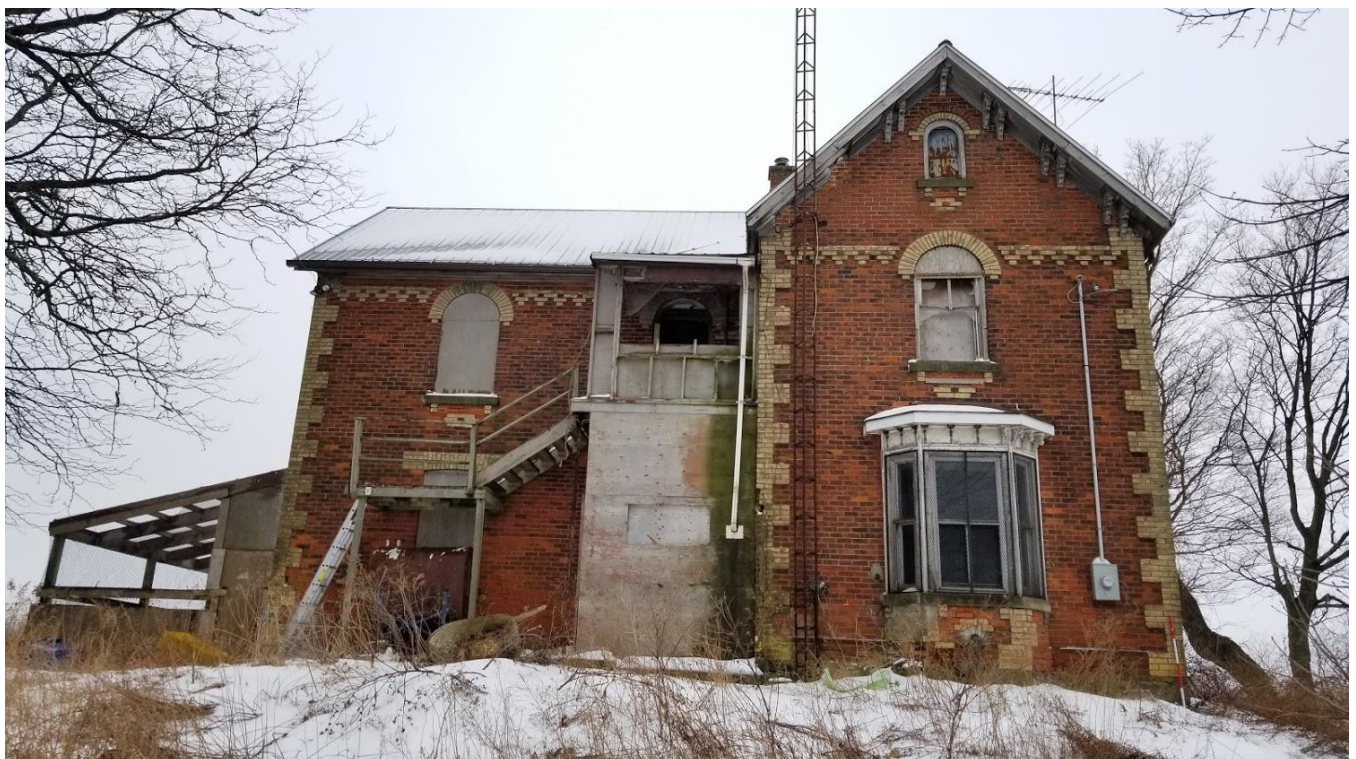
Figure 85: 9285 Twenty Road West: North façade
