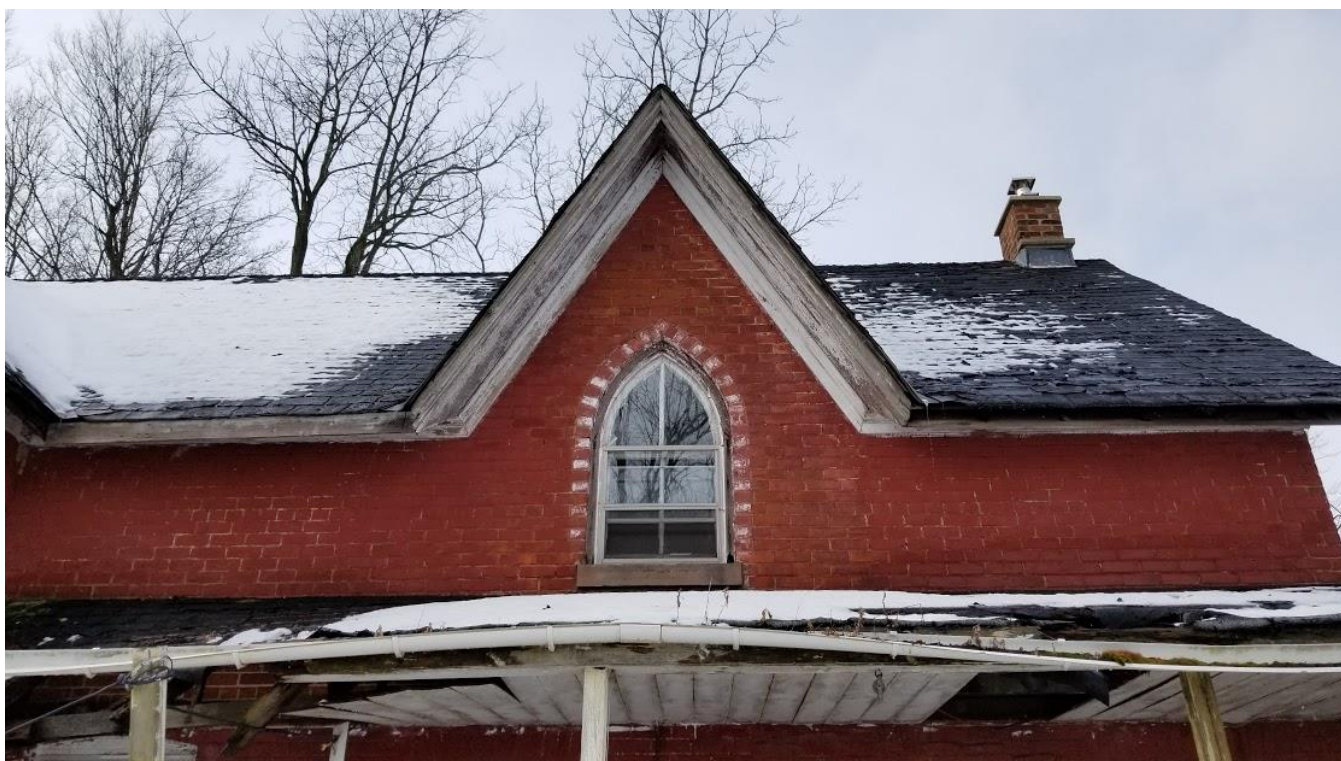
Figure 39: 9751 Twenty Road West: Cross gable on the east façade
