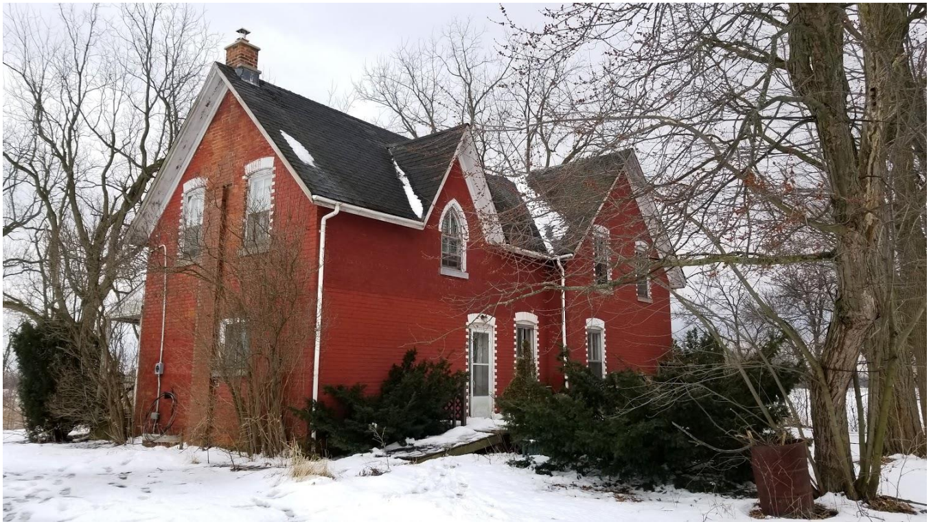
Figure 35: 9751 Twenty Road West: North and west façades
