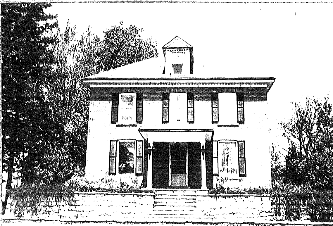
SOUTH (FRONT) VIEW ↑
