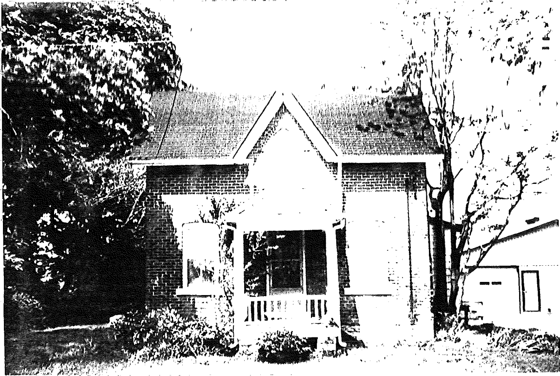
SOUTH (FRONT) VIEW ↑
