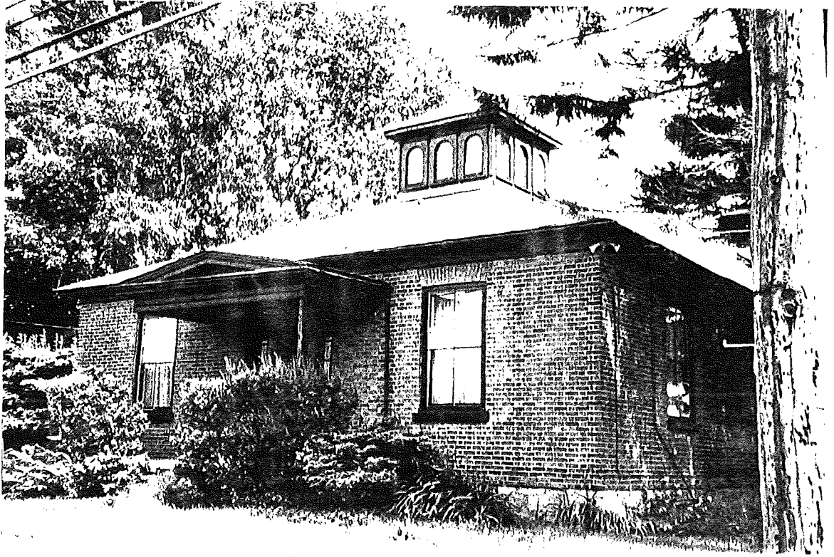
WEST (FRONT) VIEW ↑
