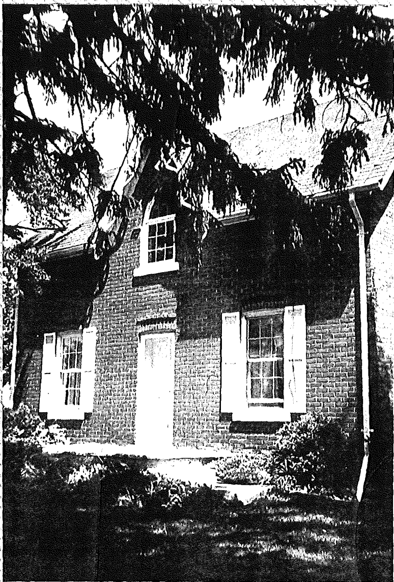
WEST (FRONT) VIEW ←
