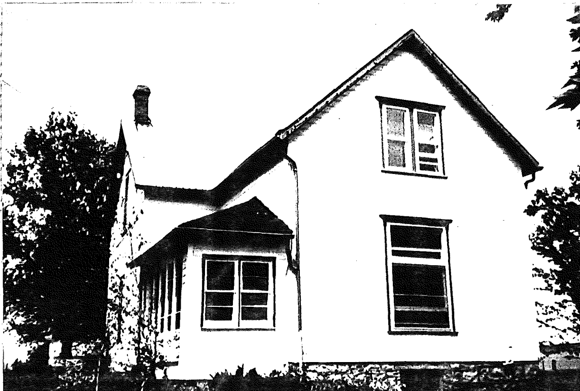
SOUTH (FRONT) VIEW ↑
