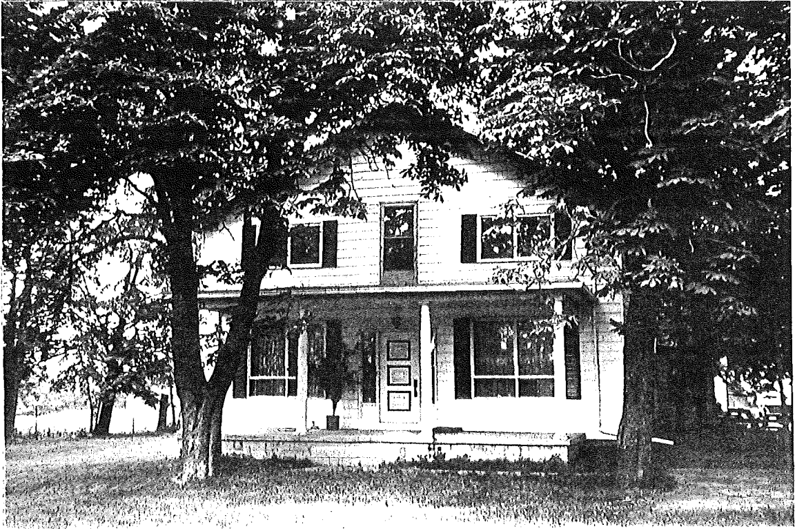
WEST (FRONT) VIEW ↑
