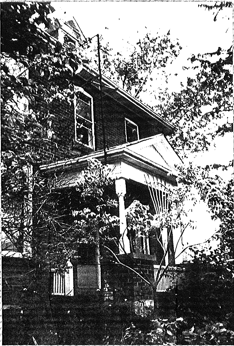
NORTH (FRONT) VIEW ←
