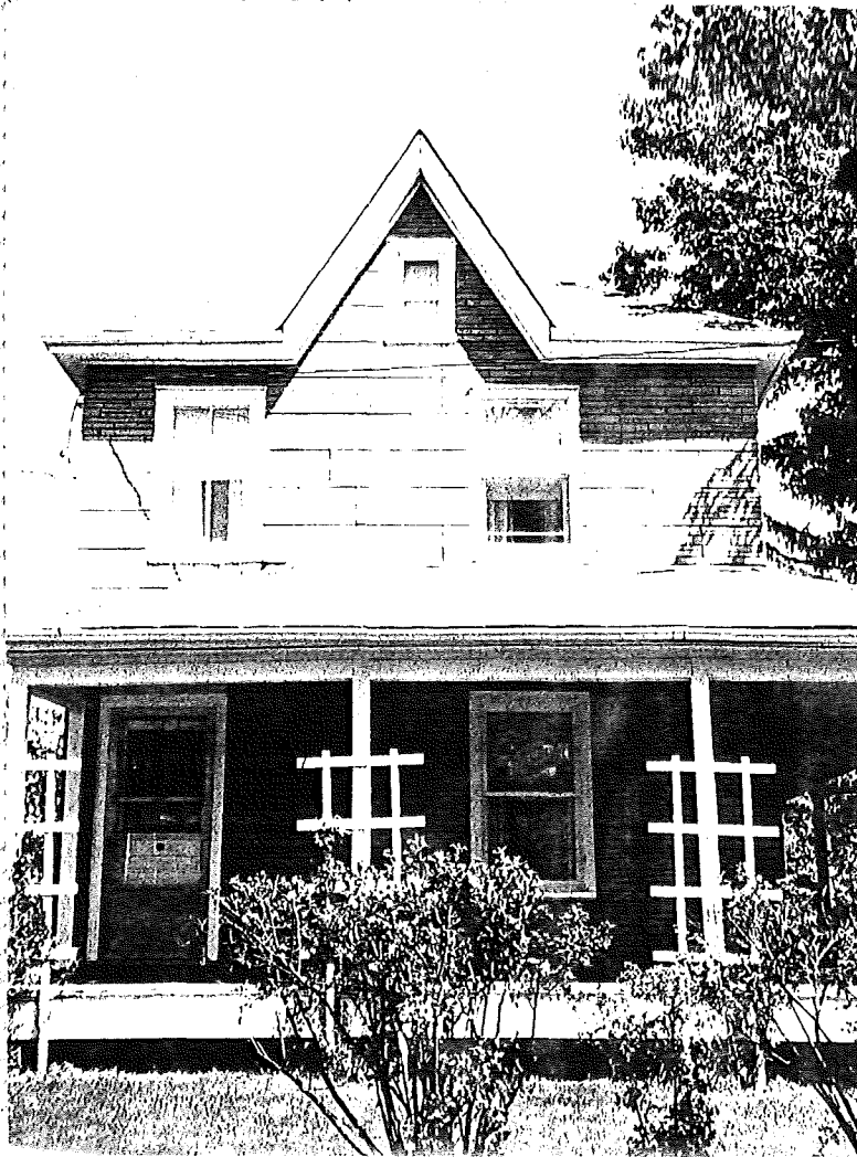
WEST (FRONT) VIEW ←
