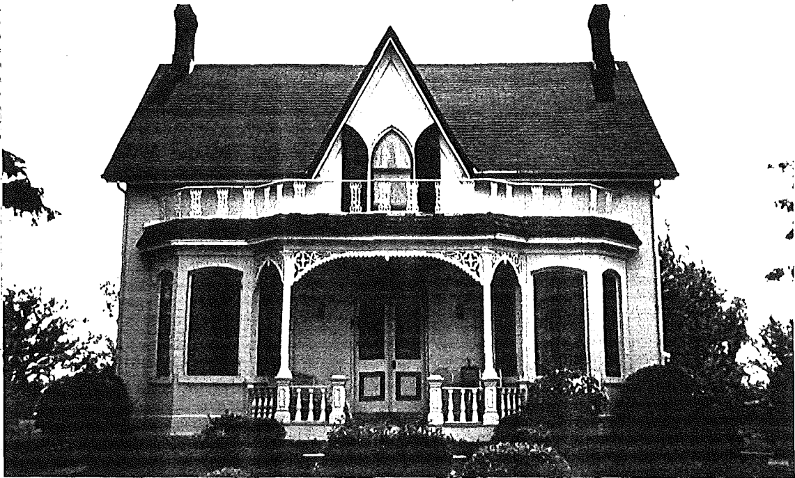
NORTH (FRONT) VIEW ↑
