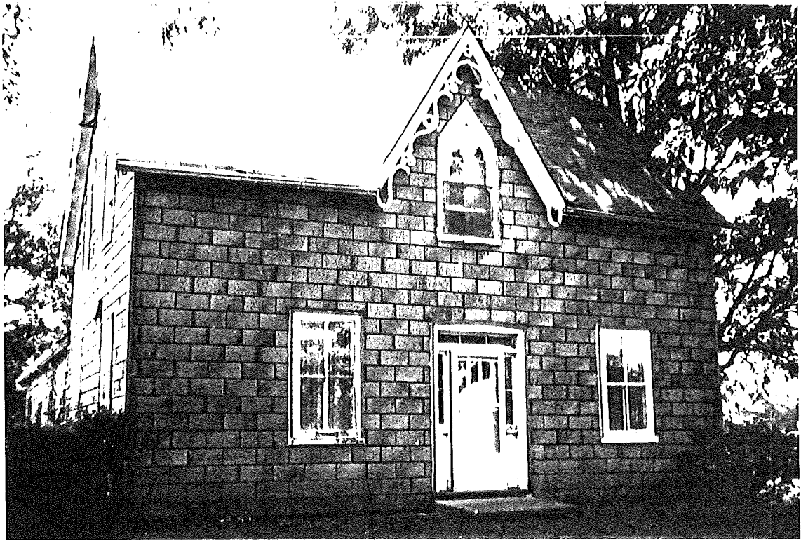
NORTH (FRONT) VIEW
