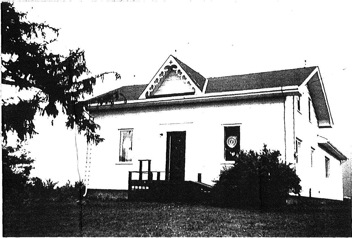
NORTH (FRONT) VIEW ↗
