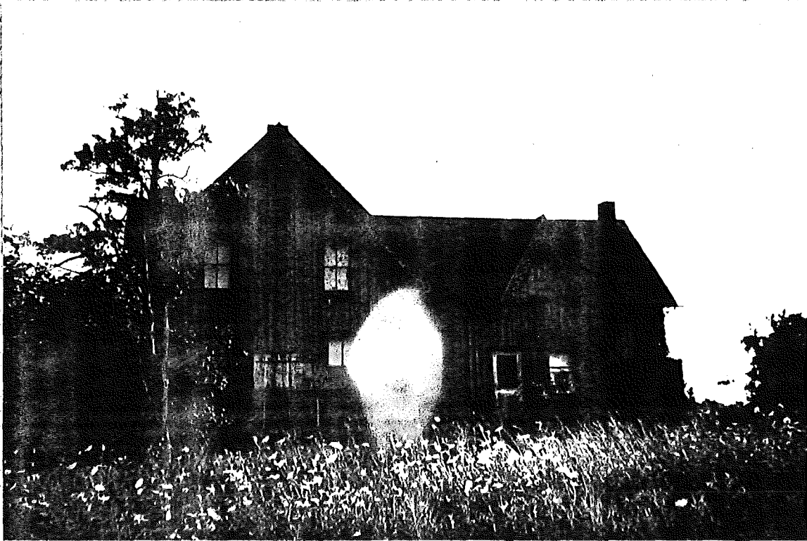
NORTH (FRONT) VIEW ↑
