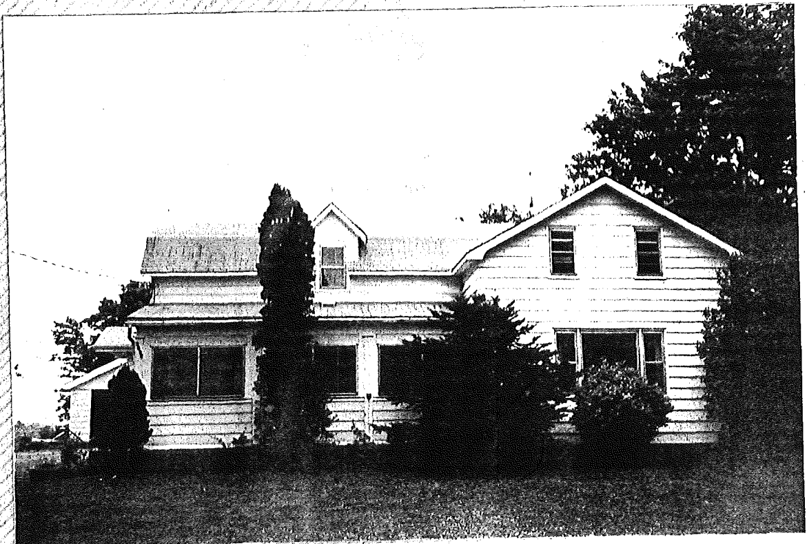
NORTH (FRONT) VIEW
