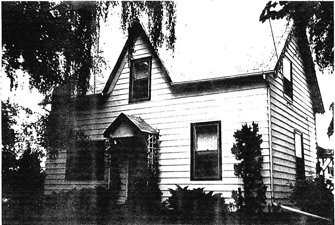
SOUTH (FRONT) VIEW ↑
