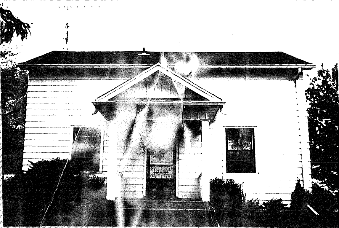
WEST (FRONT) VIEW ↑
