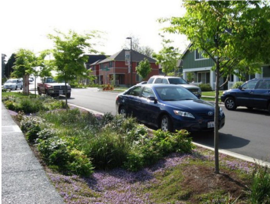
Figure 8: LID BMP Conveyance Swale
