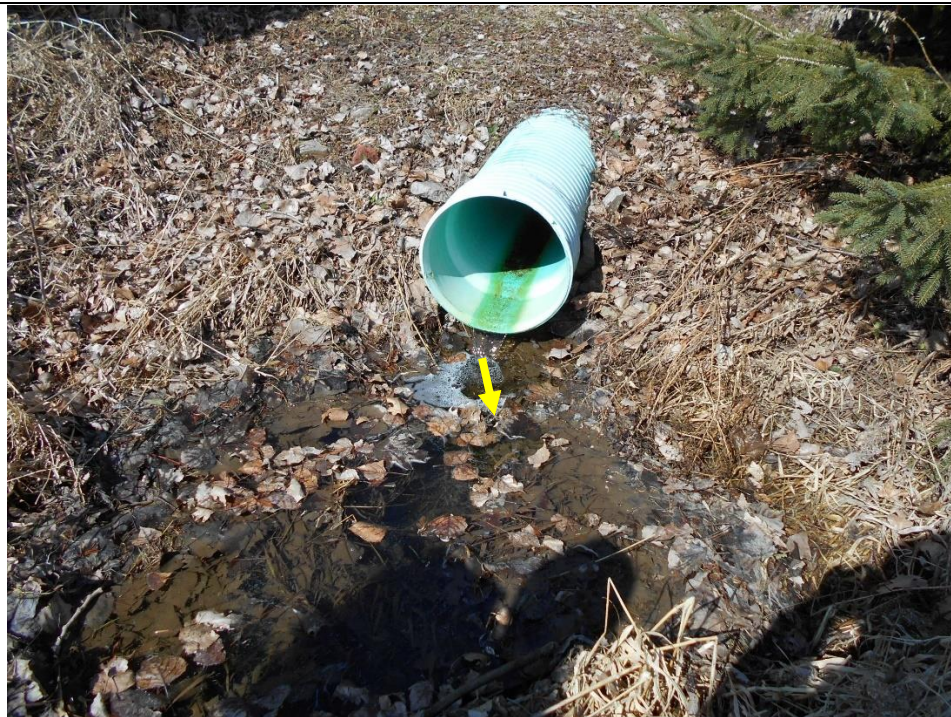
The feature originated at a culvert and was poorly defined.
