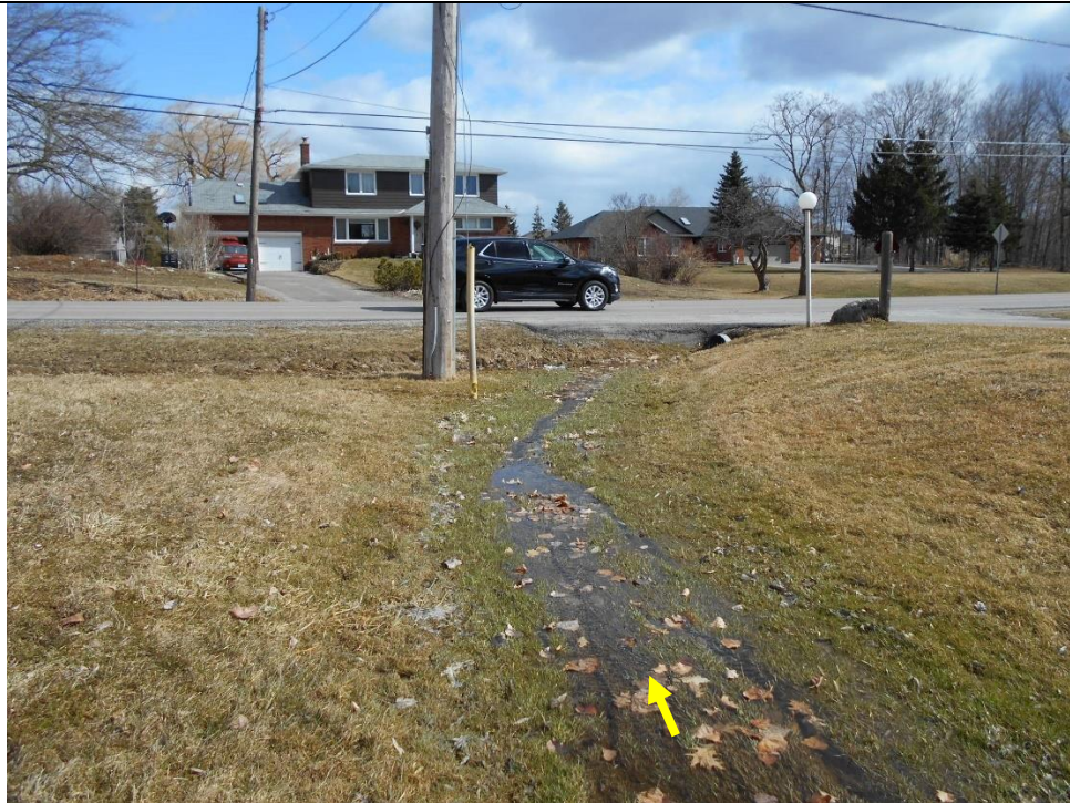
The feature lacked bed and bank definition and conveyed flows towards a roadside ditch at Twenty Road West.
