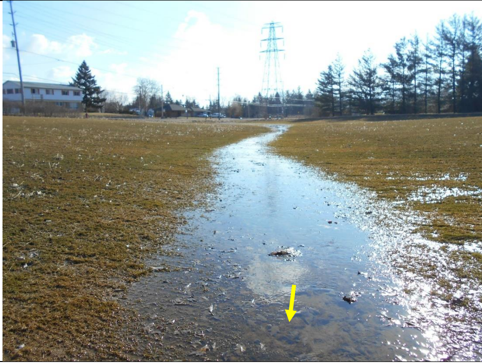
The feature lacked channel definition and conveyed flows through an agricultural field.
