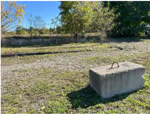
Grid A-2 view from West side looking SE
