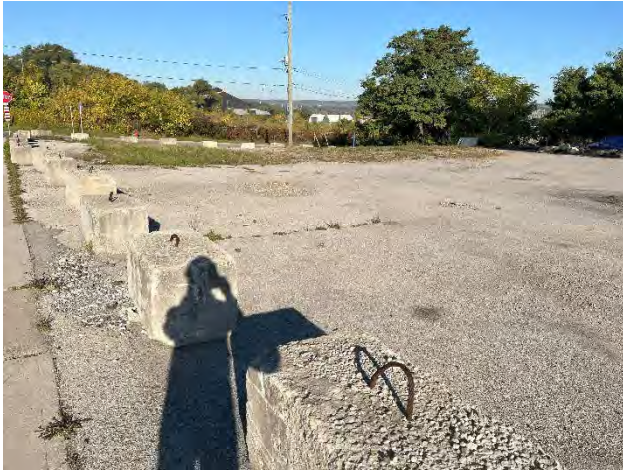
Grid A-1 view from SE corner looking West
