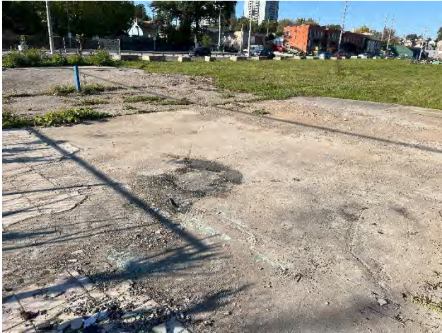
Grid C-1 view from NE corner looking SW
