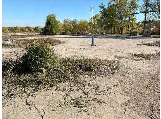
Grid C-2 view from SW corner looking NE
