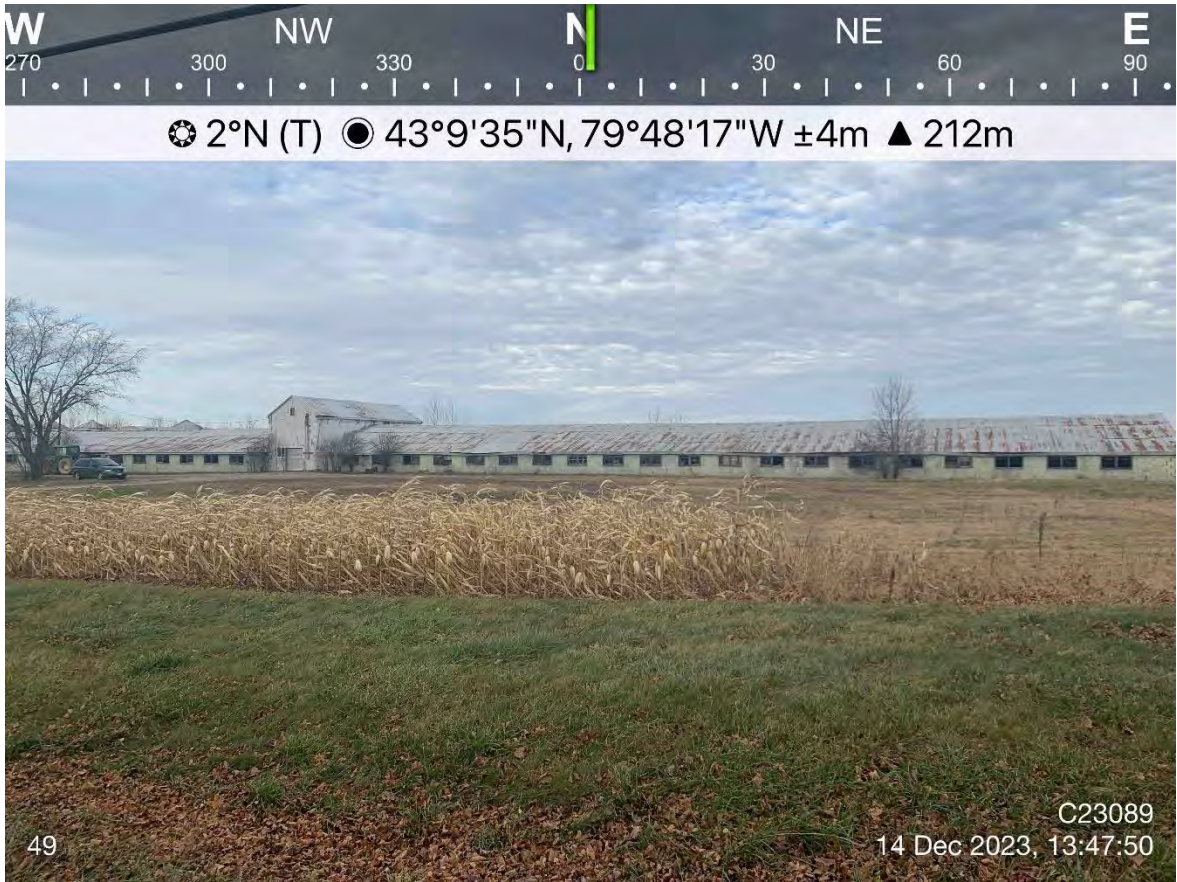
Photo 5: Operation #49 – Remnant farm showing barn in poor condition.
