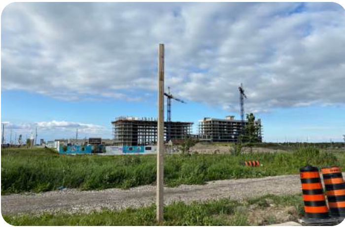
Midrise development underway adjacent to the heritage greene shopping centre
