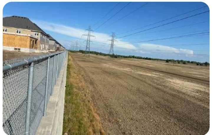
The north side of the subject site is lined by the hydro corridor and a large retaining wall along existing residential development
