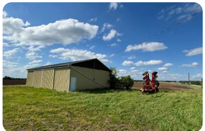
Various agricultural structures are located throughout the subject site such as this barn
