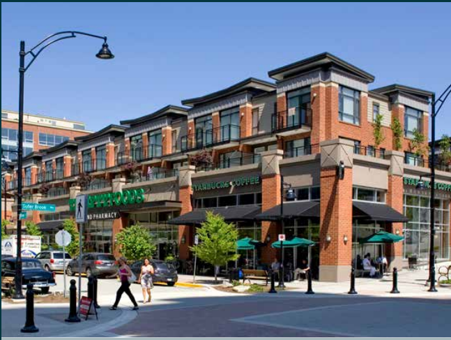
Fig. 4.3.2a - Image example of corner building with façades that appropriately address both street frontages.
