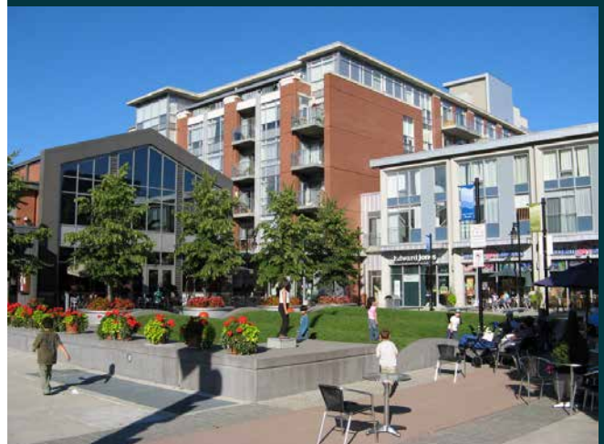
Fig. 4.2.4h - Image example of urban square bordered by mixed-use built form, with opportunities for flexible programming.
