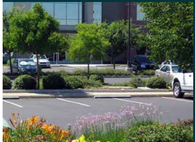
Fig. 4.5.4 - Image example of expansive surface parking divided into smaller parking areas through use of landscaping.
