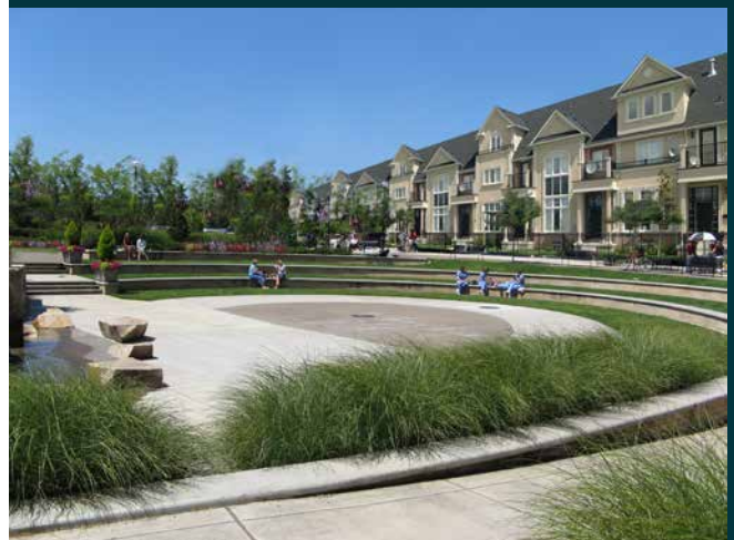
Fig. 4.2.4i - Image example of urban square with informal seating, bordered by compact built form.
