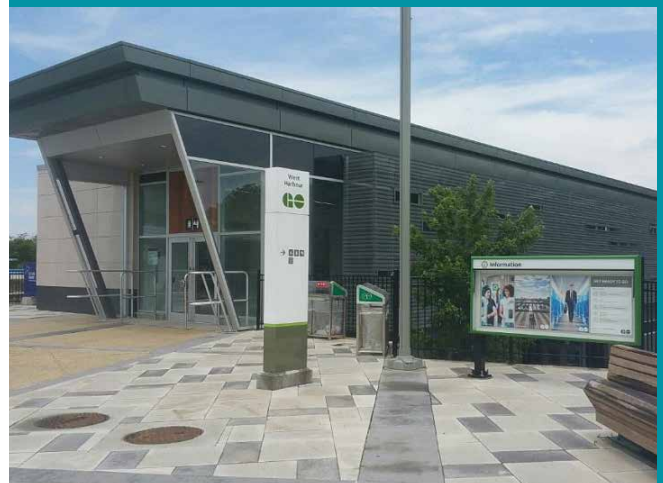
Fig. 2.2.1b - Downtown Hamilton's West Harbour Go Station to be connected to subject lands via Upper James Street BRT.
