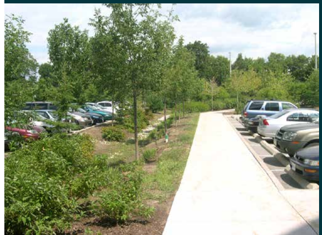
Fig. 4.1.2f - Image example of parking area integrating a bioswale and pedestrian walkway.
