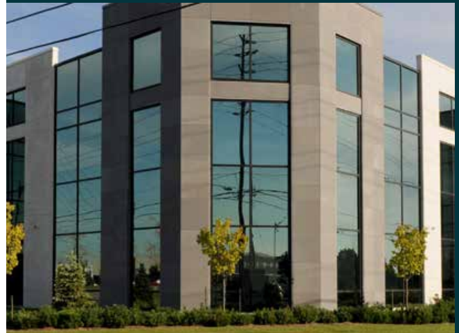
Fig. 4.4.2a - Image example of an office employment building oriented toward prominent corner location.
