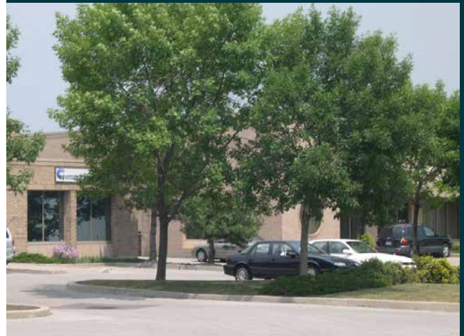
Fig. 4.5.3 - Image example of office building with windows facing the street and setbacks to accommodate parking and landscaping.
