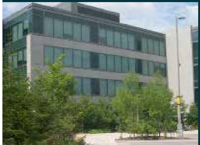
Fig. 4.4.5 - Image example of rooftop mechanical equipment screened from ground level view through integration with roof form.
