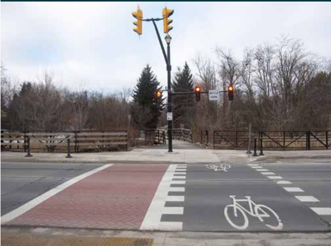
Fig. 4.2.2d - Image example of signalized crosswalk at mid-block trail crossing.
