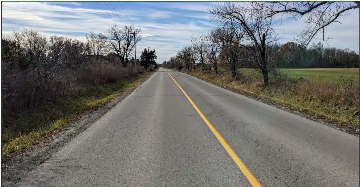
Photo 7: View looking west along White Church Road East.
