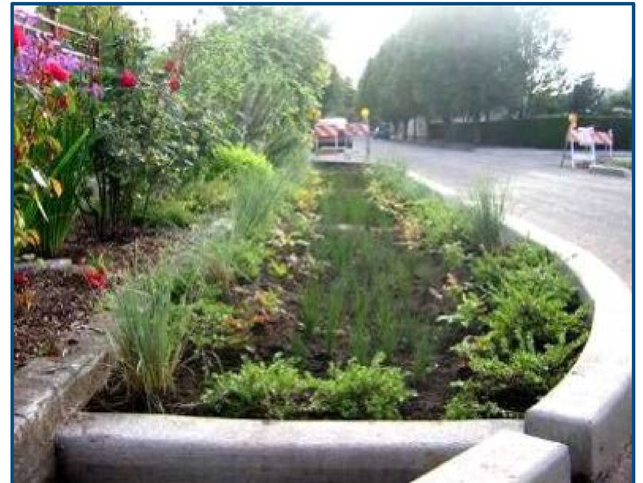
Example of Bioretention Area. Source: City of Portland, BES.
