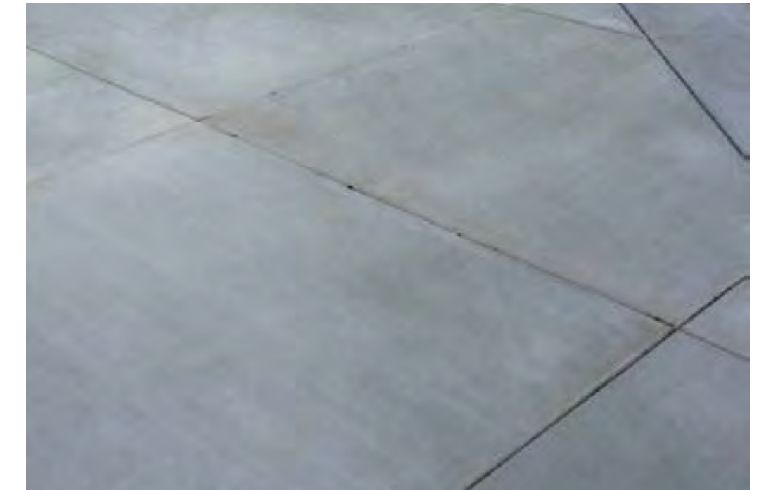
05 CONCRETE WITH GEOMETRIC SAW-CUT MOSAIC
