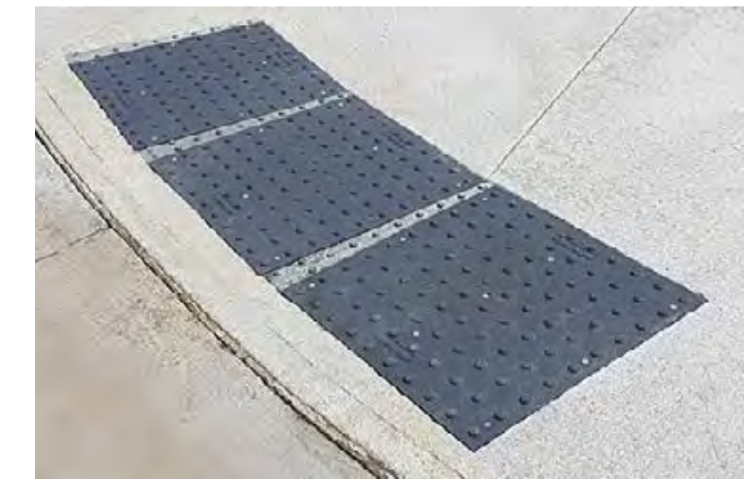
02 AODA COMPLIANT DROP CURB AND TACTILE INDICATORS
