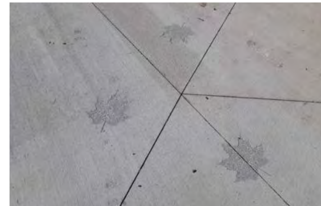
05 CONCRETE WITH SANDBLASTED ESCARPMENT LEAF MOSAIC
