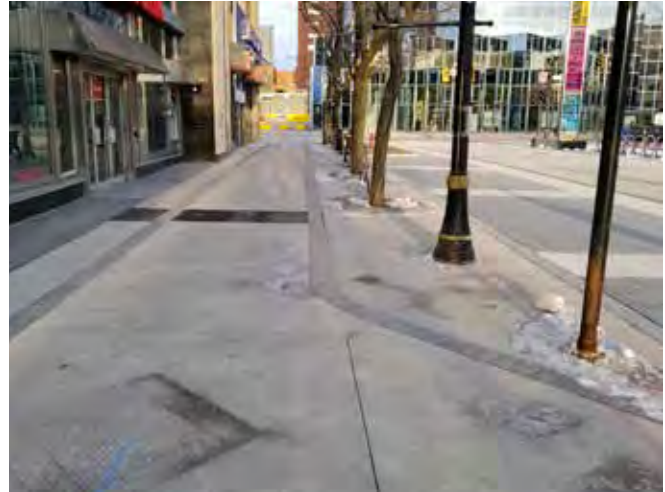
Figure 3: Urban Braille - Pedestrian Clearway with Shoreline and Diamond Marker
