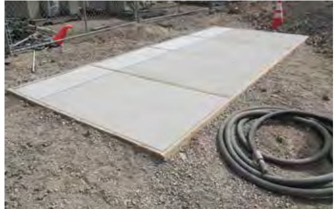
Figure 6: Trial Run "Mock Up" of Concrete Patterning Process
