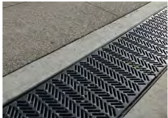
Figure 7: Vehicular Drive Lane with Integrated Trench Drain
