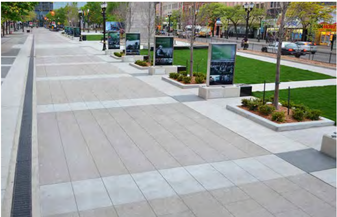
Figure 2: The Gore Pedestrian Promenade. A combination of smooth finished bands and soft finished fields.
