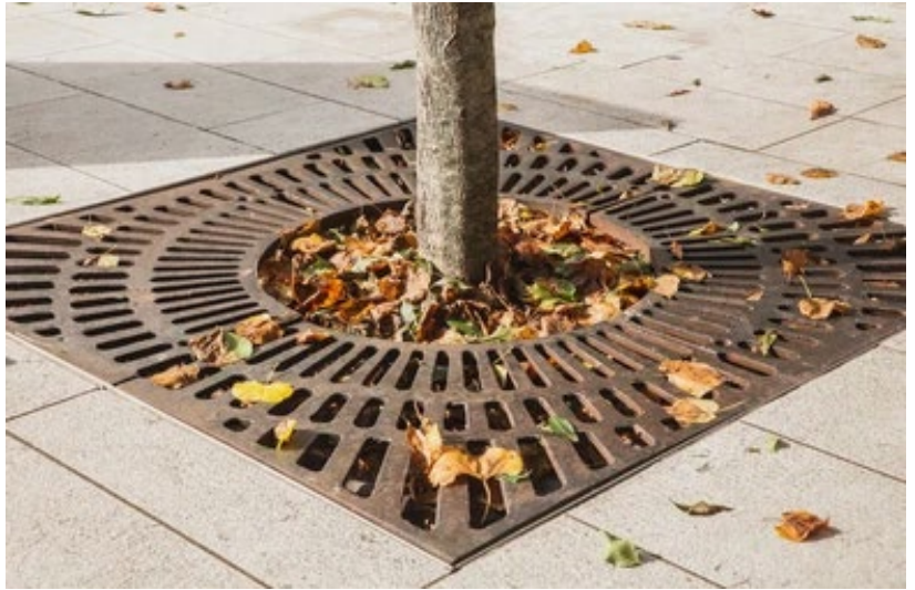
Figure 7: Tree grate with large inner ring and square outer perimeter.
