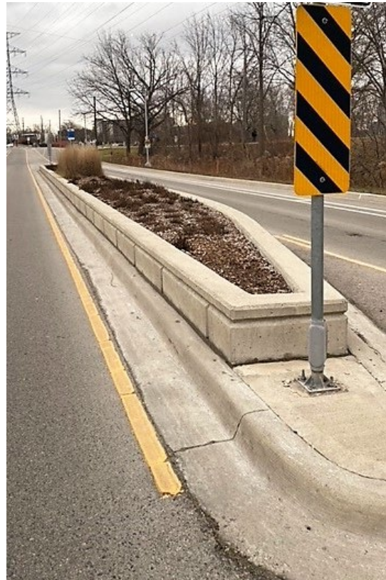
Figure 1: Example of raised traffic island.
