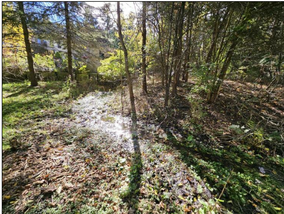
Photo 13. The SCT1-3 feature draining northwards from the armourstone wall. Good flow observed on October 16, 2024.
