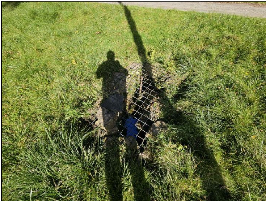
Photo 15. Open grate observed along the SCT1-3 subsurface drainage pathway. Standing water observed on October 16, 2024.
