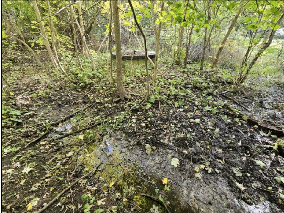
Photo 14. Feature SCT6 arising from a groundwater seep near an old well structure. Minimal flow observed on October 16, 2024.
