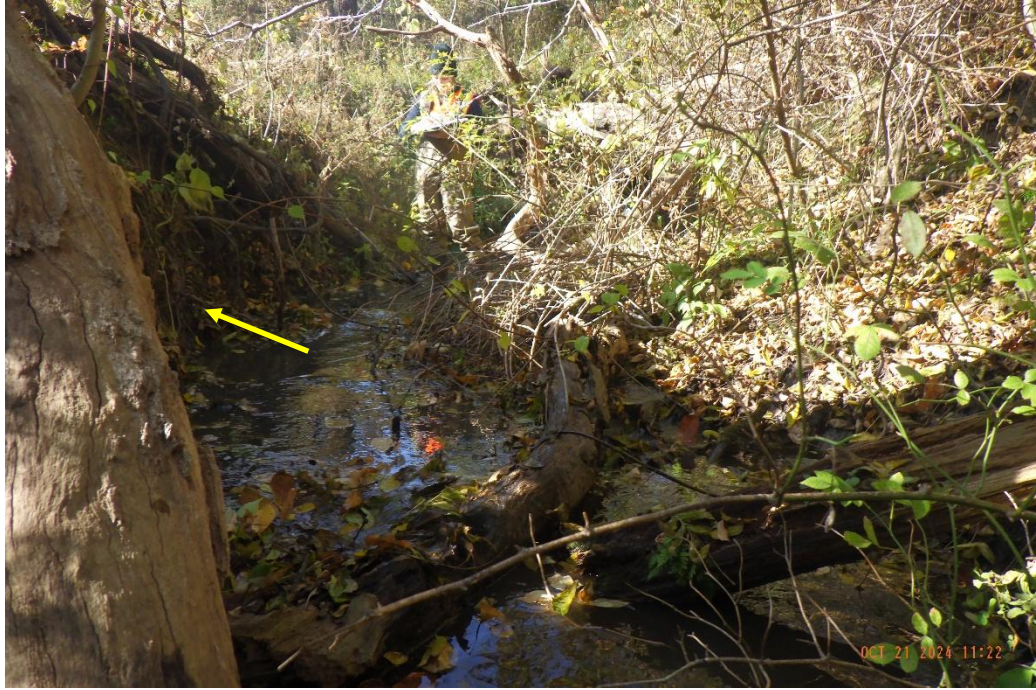
Some erosion was observed along the channel as well as in the scour pool (yellow arrow – general bank erosion).
