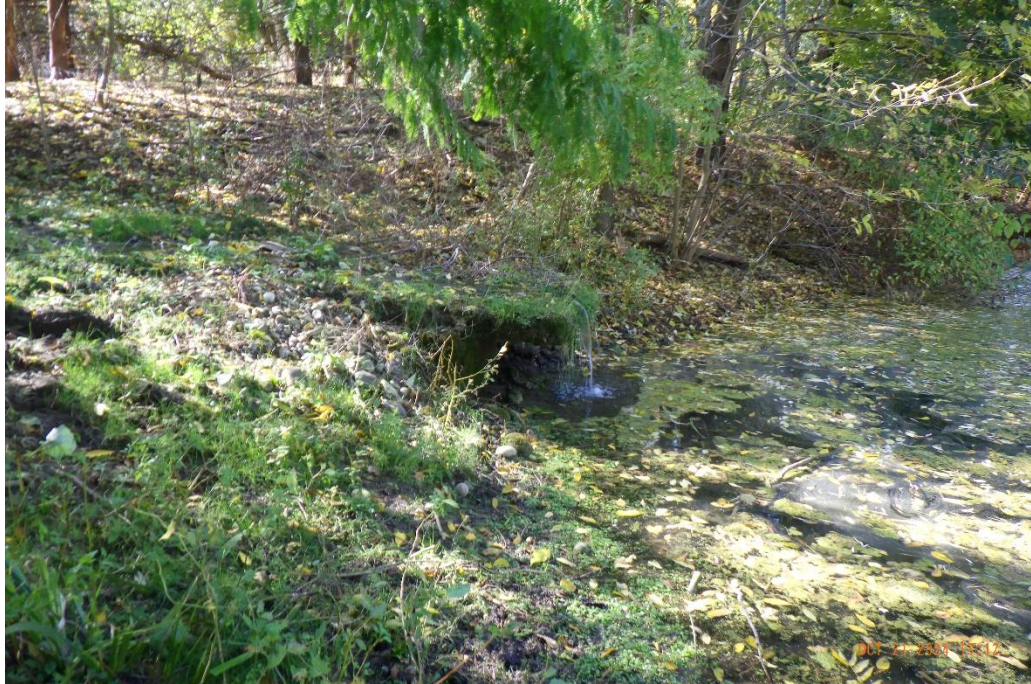
The drainage feature was observed to enter the pond via overland flow over a concrete slab.
