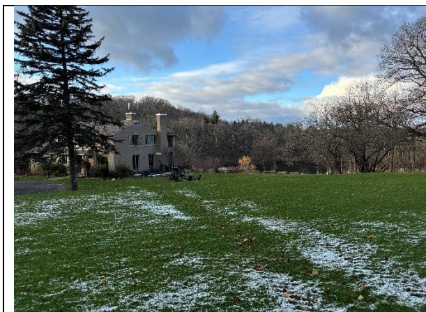
Image 7: Residential house, facing west
