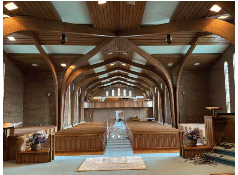
Interior View of 1570 Main Street W (Binkley United Church) Source: ATA Architects Inc. (2024)
