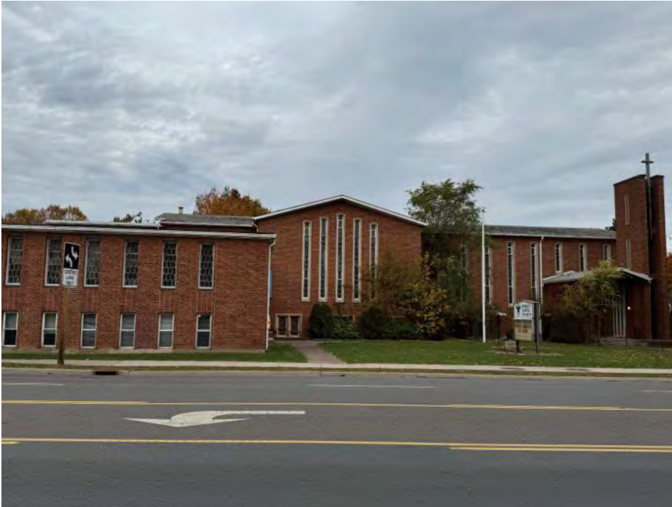
Exterior View of 1570 Main Street W (Binkley United Church) Source: ATA Architects Inc. (2024)
