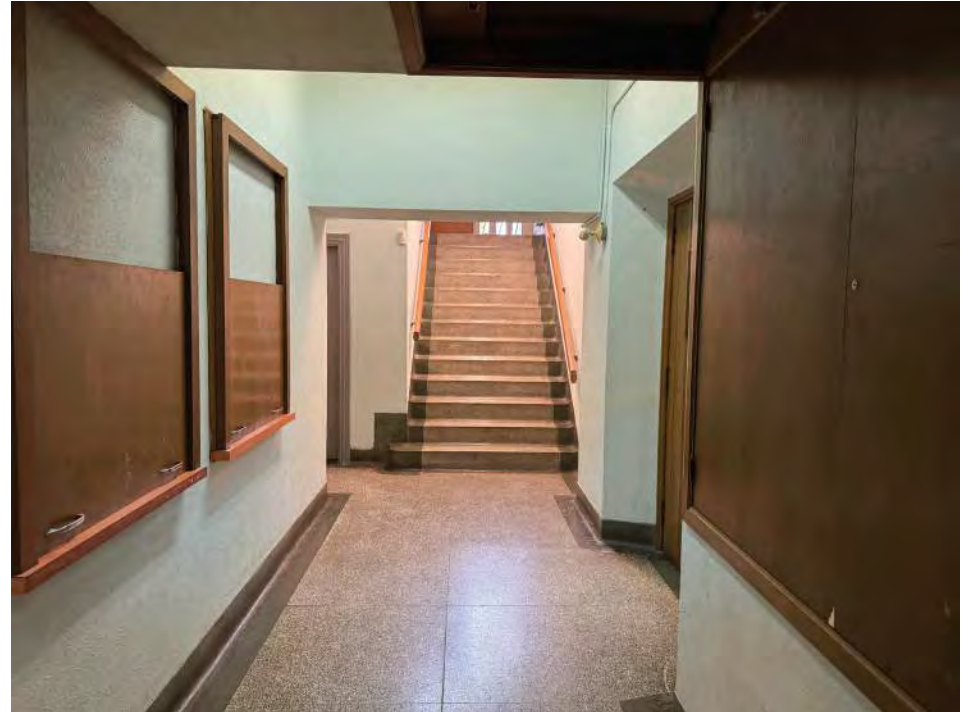
Interior View of 1570 Main Street W (Binkley United Church) Source: ATA Architects Inc. (2024)
