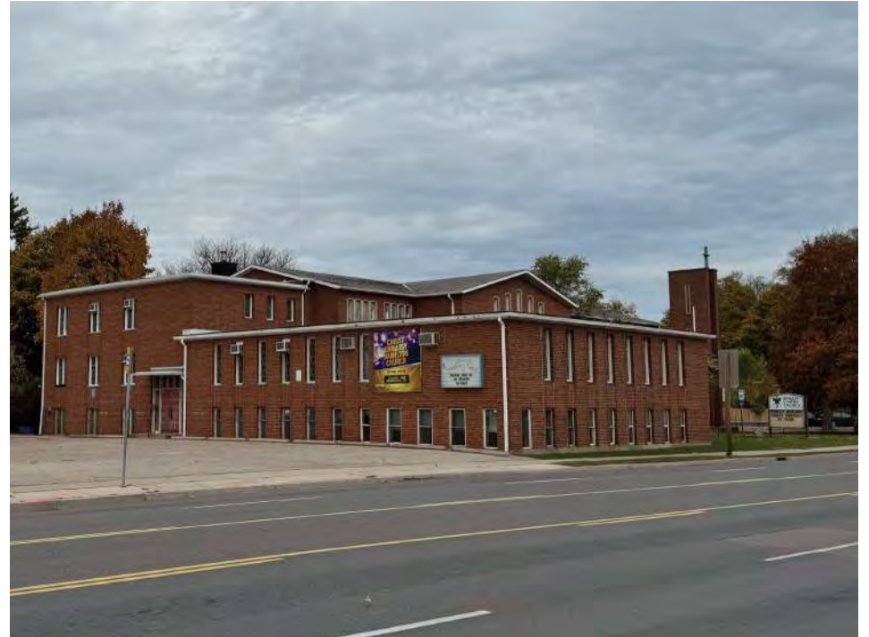
Exterior View of 1570 Main Street W (Binkley United Church) Source: ATA Architects Inc. (2024)
