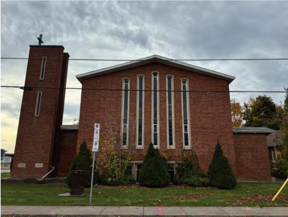
Exterior View of 1570 Main Street W (Binkley United Church) Source: ATA Architects Inc. (2024)
