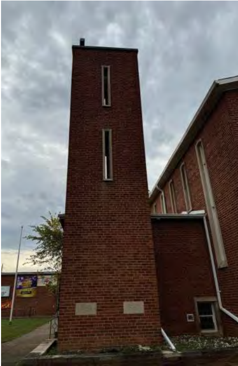
Exterior View of 1570 Main Street W (Binkley United Church) Source: ATA Architects Inc. (2024)
