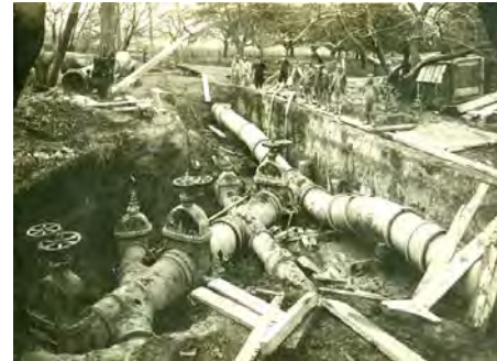
Laying early water mains in Hamilton
