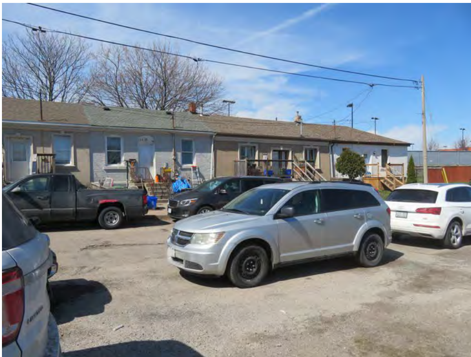
CATHCART STREET – the north end of the street dead ends at the developmetn site – 1-storey row
