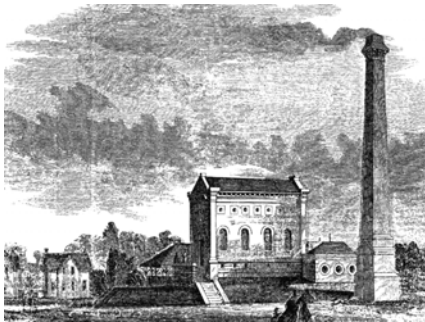
Pumphouse at the Hamilton Waterworks, 1859
