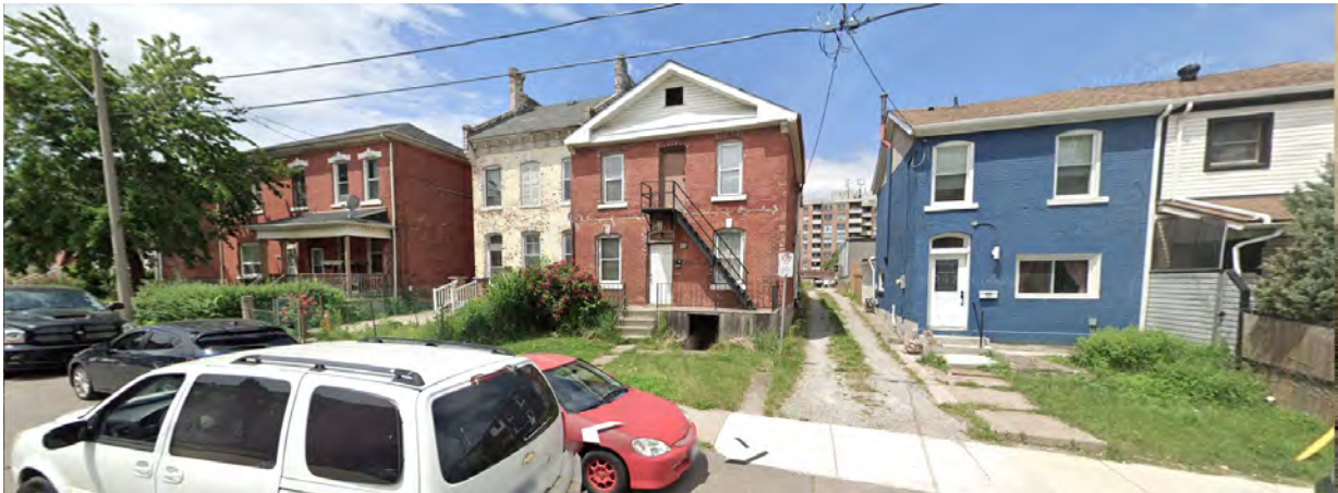
CATHCART STREET, west side - 2-storey 19 th century dwellings
