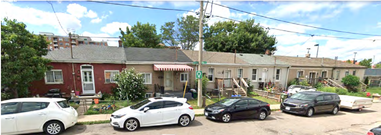
CATHCART STREET, west side – 19 th century row of workers' cottage
