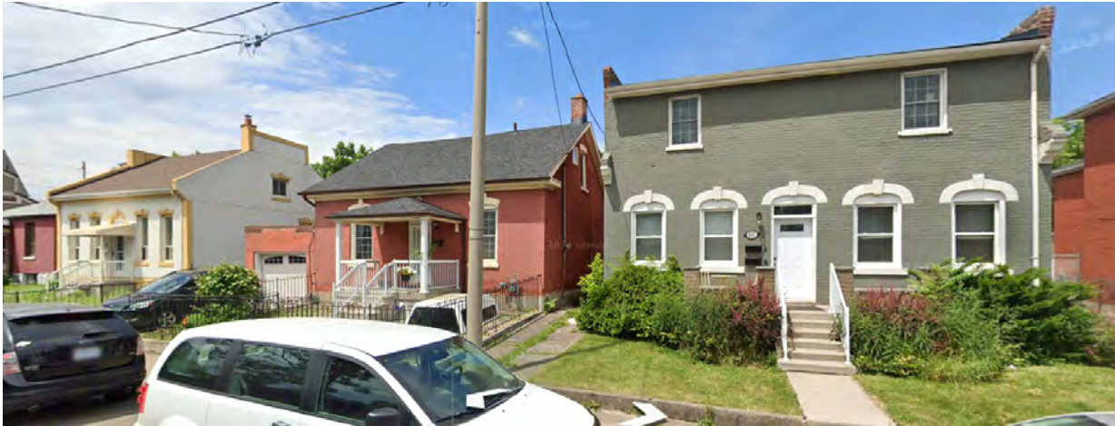
CATHCART STREET, west side – 1 and 2-storey 19 th century dwellings
