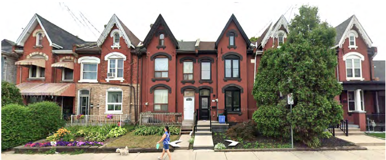
WELLINGTON STREET NORTH, east side – 2.5-storey Victorian rows with side gables
