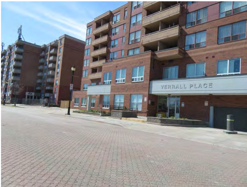
VERRALL PLACE – recent residential development across the street on Ferguson Avenue North – 6-8 storeys in height
