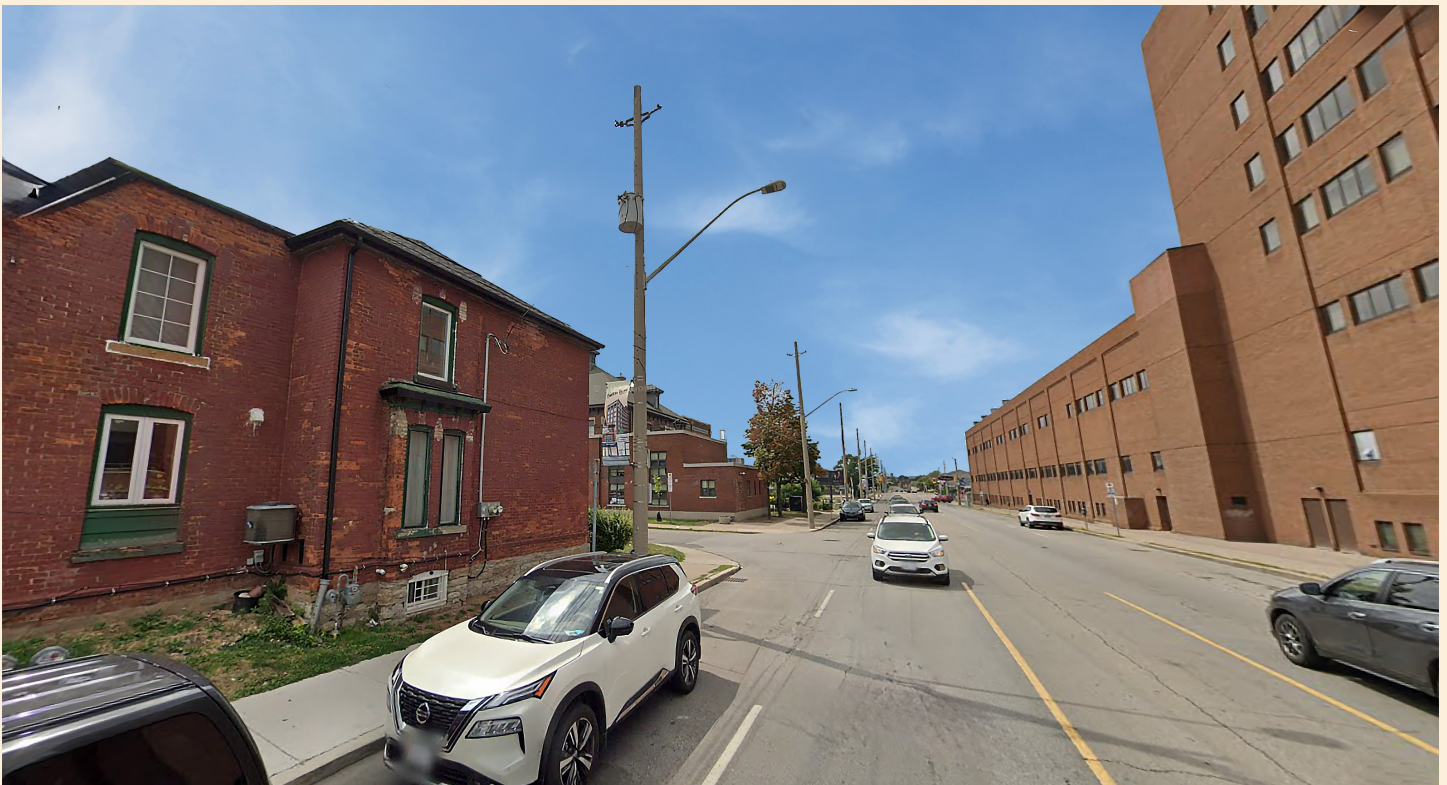
View 3- Existing Condition
