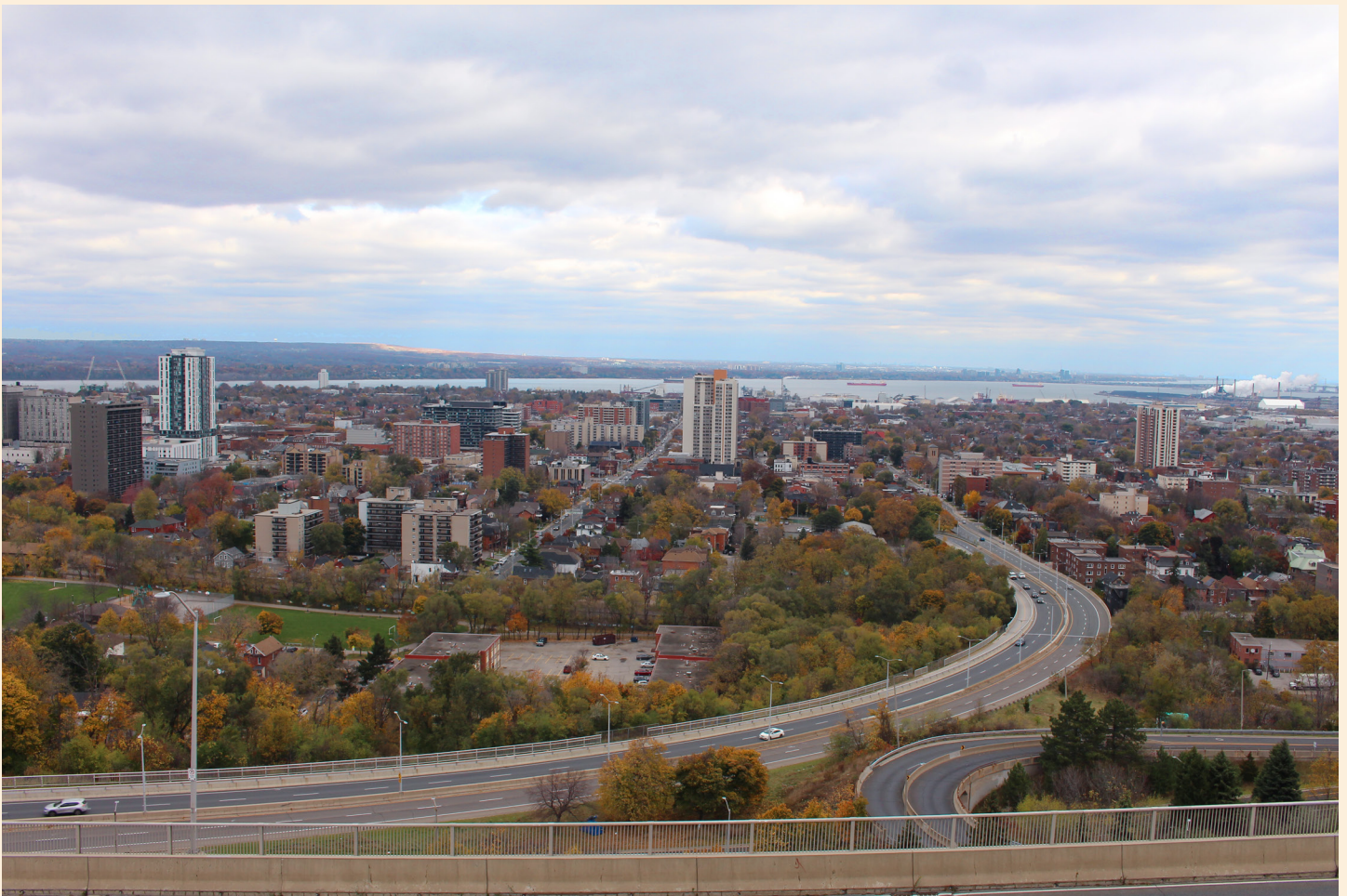
View 5- Existing Condition
