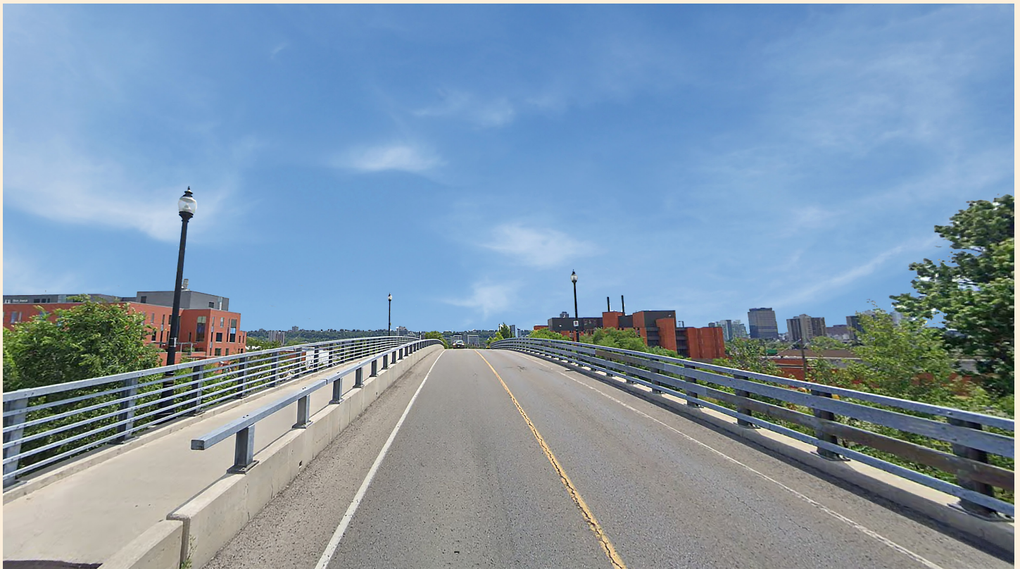
View 4- Existing Condition
