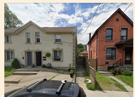
Robert St Heritage Buildings
