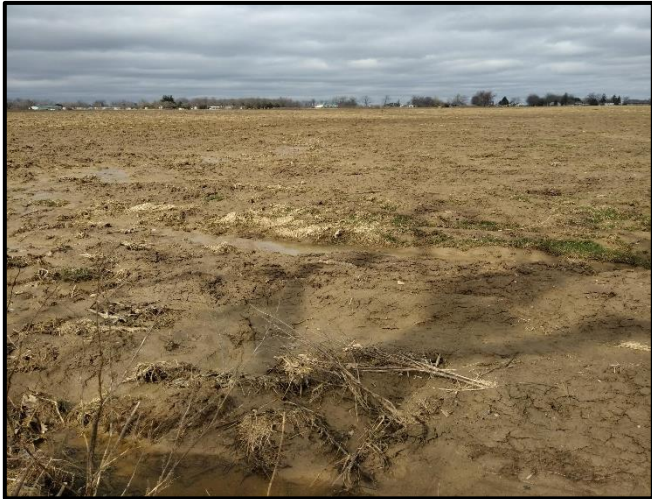
Photograph 43. Upstream View of DF16 Taken During Round 1. View: N Date Taken: March 27, 2024 Site: Parcel 2
