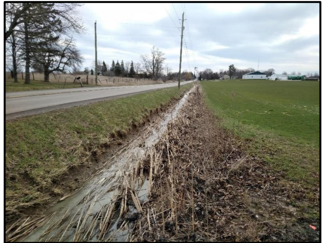
Photograph 4. Downstream View of DF2 Taken During Round 1
