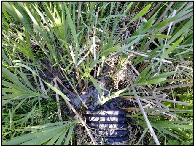
Photograph 48. Upstream View of Flow Entering Culvert Associated with DF18a Taken in Round 2. View: N Date Taken: May 31, 2024 Site: Parcel 2
