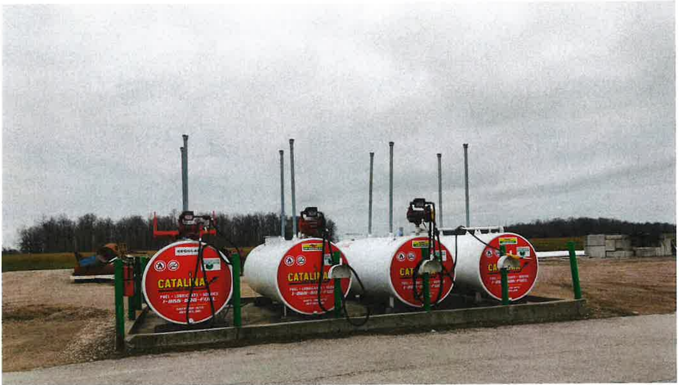
View of four (4) fuel oil ASTs located in the north-eastern portion of the subject site (looking south)
