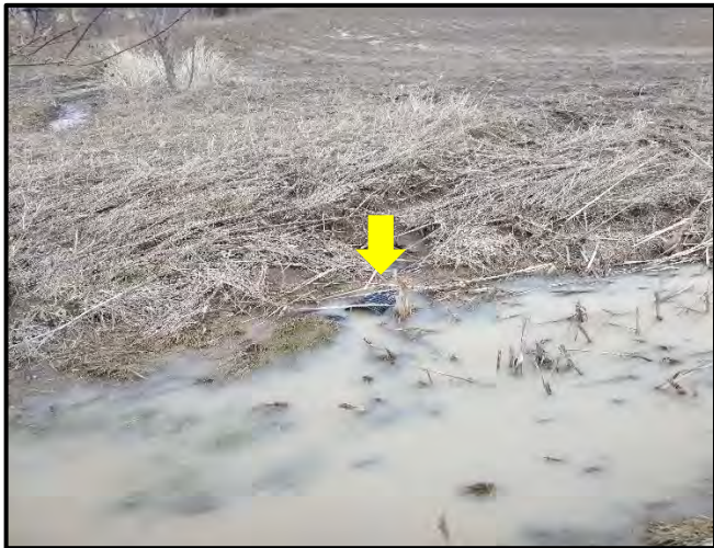
Photograph 24. Upstream View of Tile Drain Outlet (arrow) Associated with DF7 Taken During Round 1. View: N Date Taken: April 6, 2023 Site: Parcel 10
