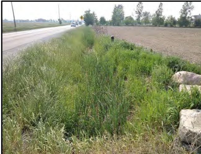
Photograph 26. Downstream View of the White Church Road Drainage Ditch. No Flow Was Observed During the Round 2 Assessment. View: W Date Taken: June 6, 2023 Site: Parcel 10
