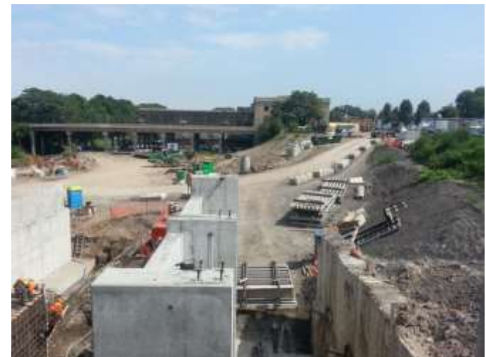
James Street North GO Station Under Construction
