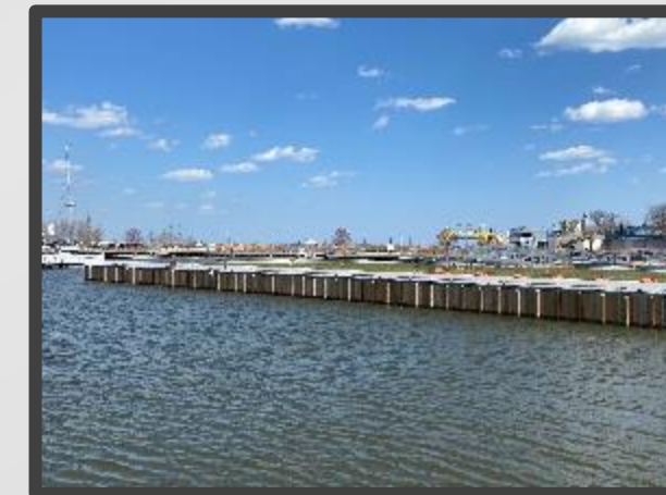
Pier 6&7 Shorewall Rehabilitation, Fish Habitat & Public Boardwalk
