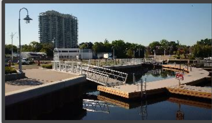
Pier 7 Shorewall, Boardwalk & Boat Slips
