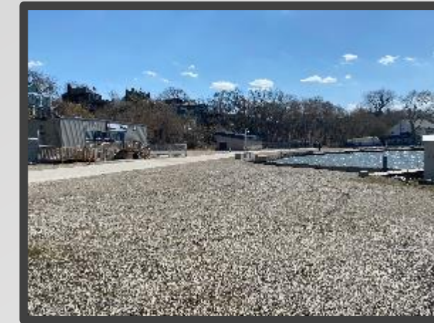
Relocation of HPS Marine Unit & Rehabilitation of former Marina
