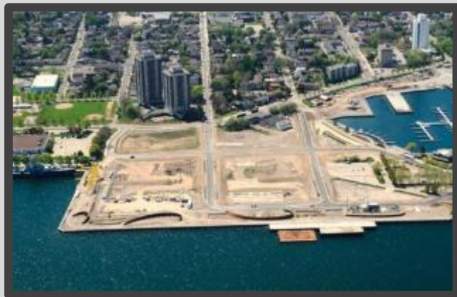
Pier 8 Servicing (Underground & Road) Infrastructure
