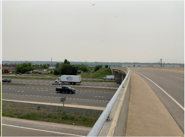
Figure 4.1: View atop Millen Rd. bridge of the QEW.
