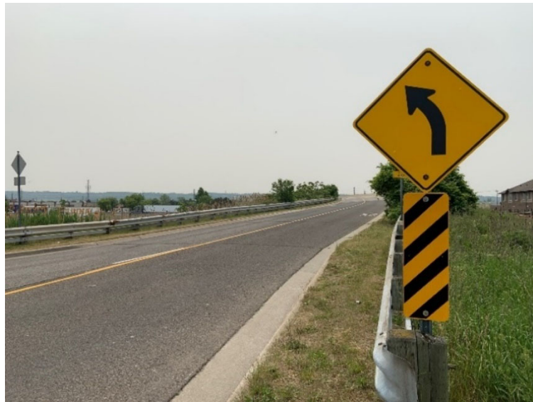
Figure 3.2: View of Millen Rd. bridge over the QEW.
